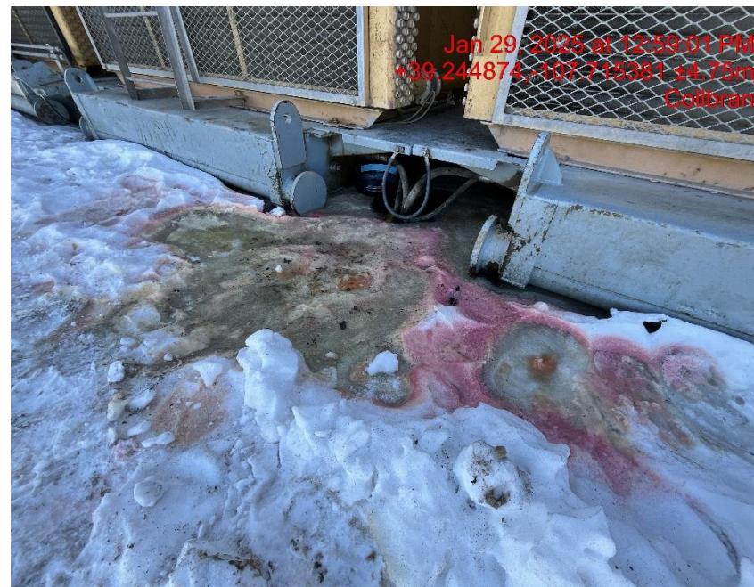
Photo # 3758 Failure to maintain chemical BMP's
