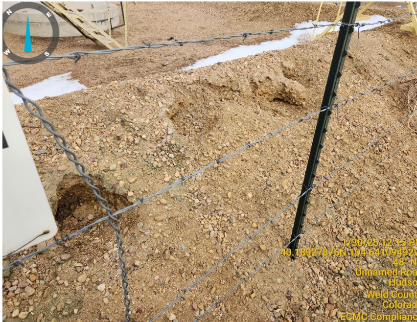
Photo 7: Holes/damage to earth berm
