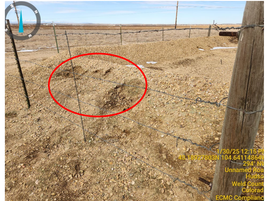
Photo 9: Holes/damage to earth berm
