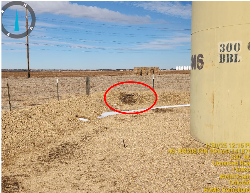
Photo 10: hole/damage to earth berm
