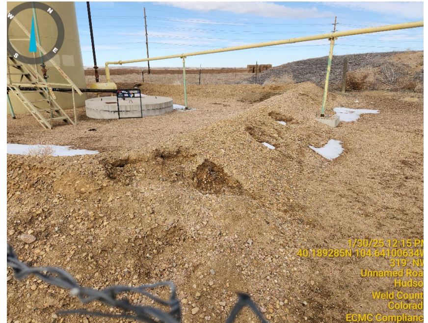
Photo 8: Holes/damage to earth berm
