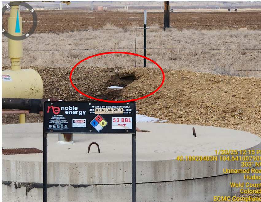
Photo 8: Hole/damage to earth berm
