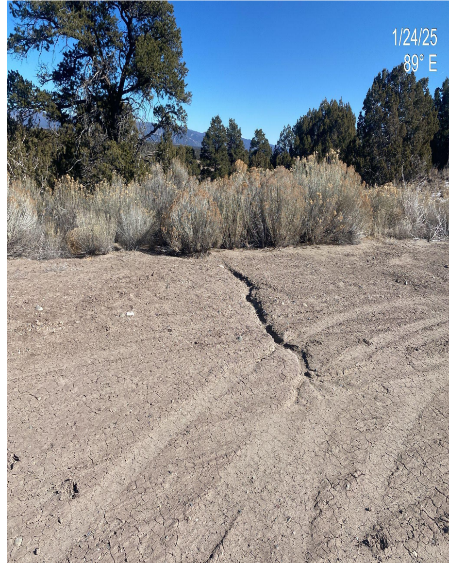
Photo 3. Rill erosion forming on the northern and eastern edges of the active pad.
