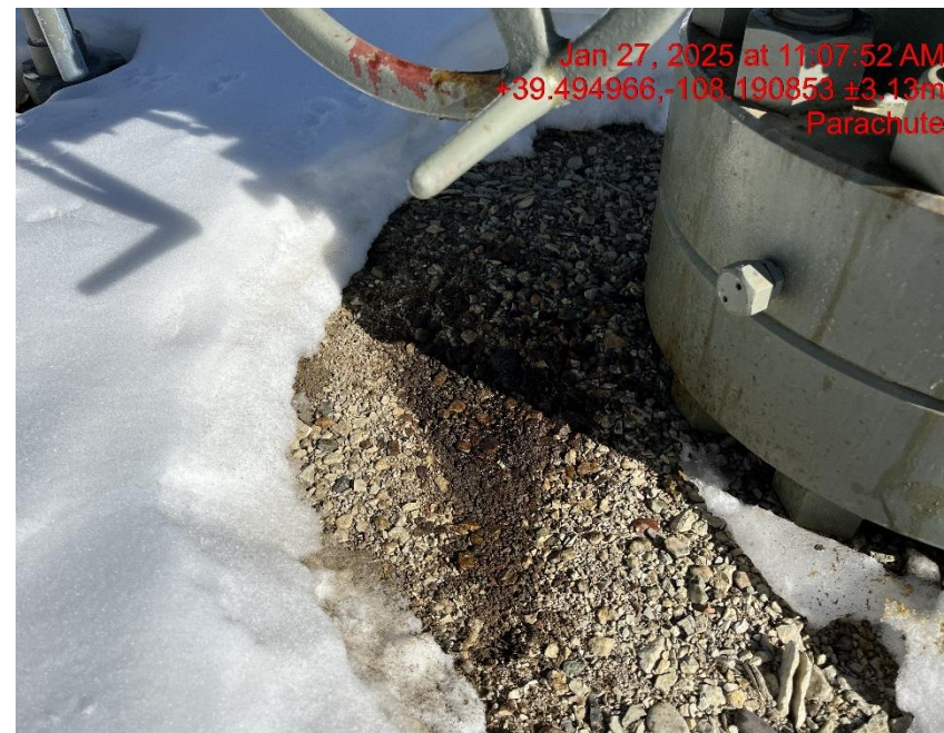
Photo # 3402 Staining around wellhead
