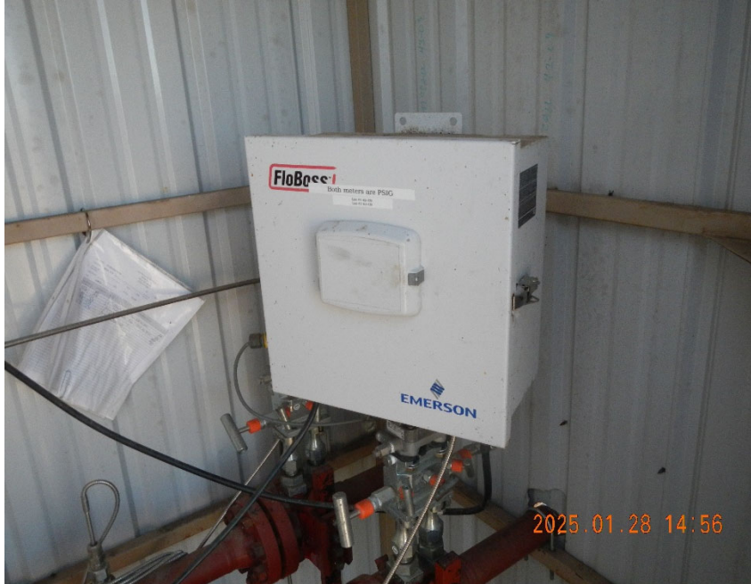
5. Gas meter inside meter shed.
