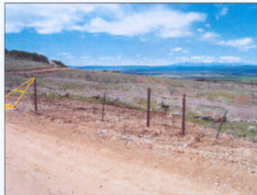
Fencing missing on north side of cattleguard 04/10/07
