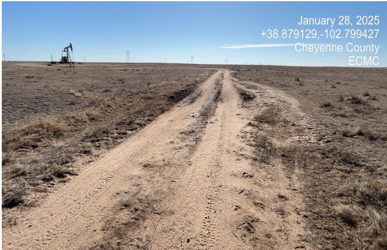
Photo 2. Facing southeast along the access road. Vehicles are causing unnecessary disturbance driving outside of the access road due to stormwater pooling on the road. The access road must be maintained and shall not drive outside of the access road boundary.
