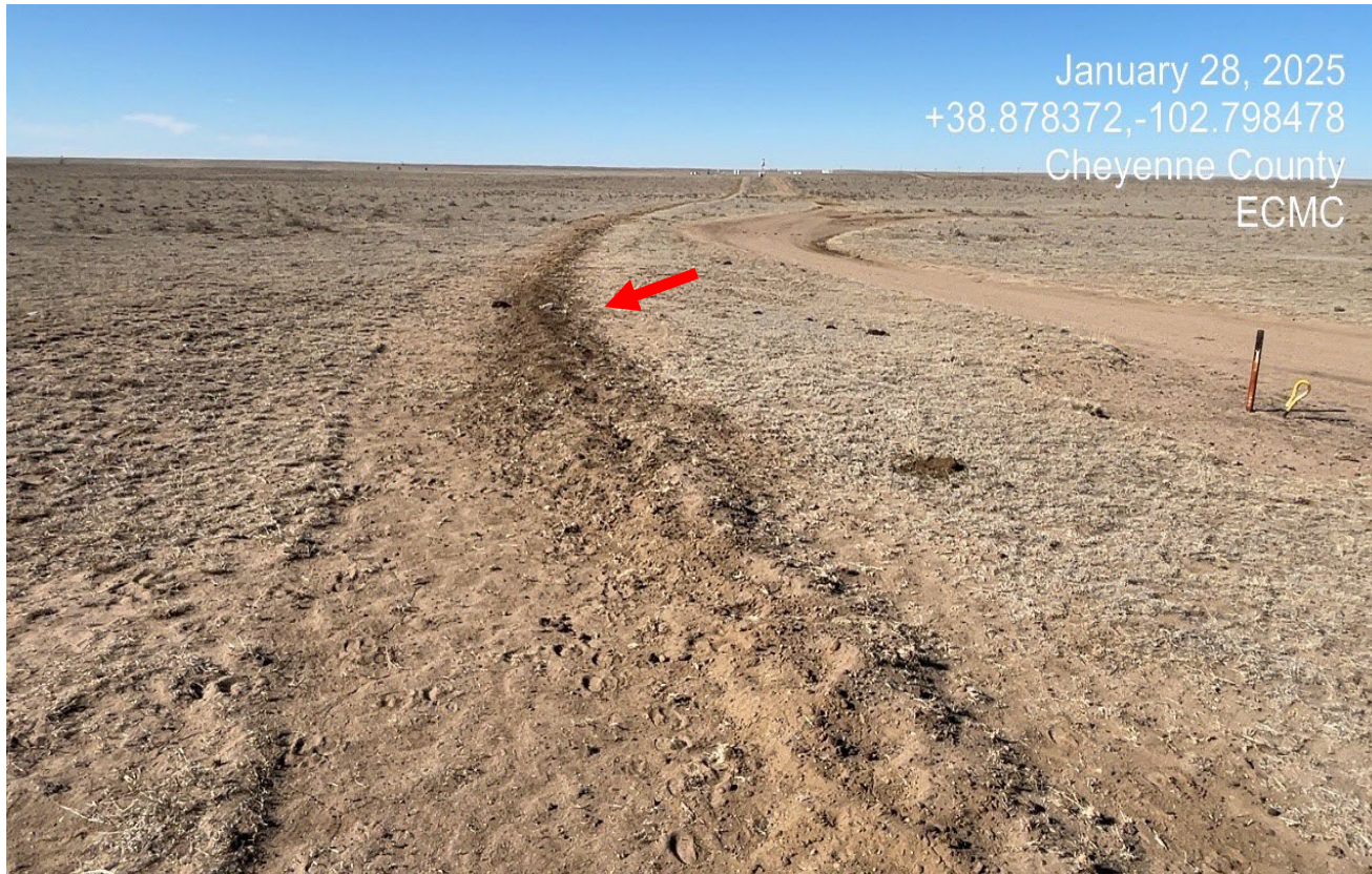
Photo 10. There has been a new electric line trenched which goes to the Rhoades Unit 5-5. The disturbed soils must be seeded and stabilized.
