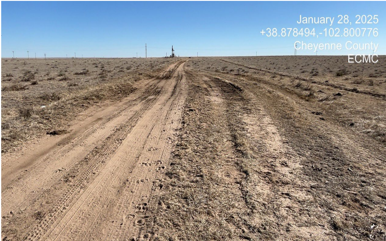
Photo 11. Facing east along the access road. Vehicles are causing unnecessary disturbance driving outside of the access road due to stormwater pooling on the road. The access road must be maintained and shall not drive outside of the access road boundary.
