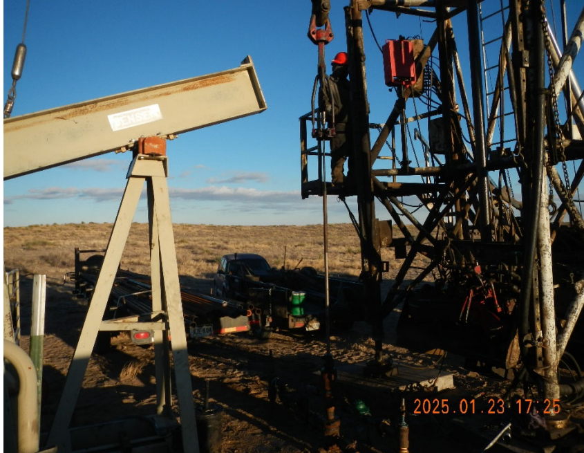
4. View of pump jack with horse head removed, Crew will be getting well set up to return to production.
