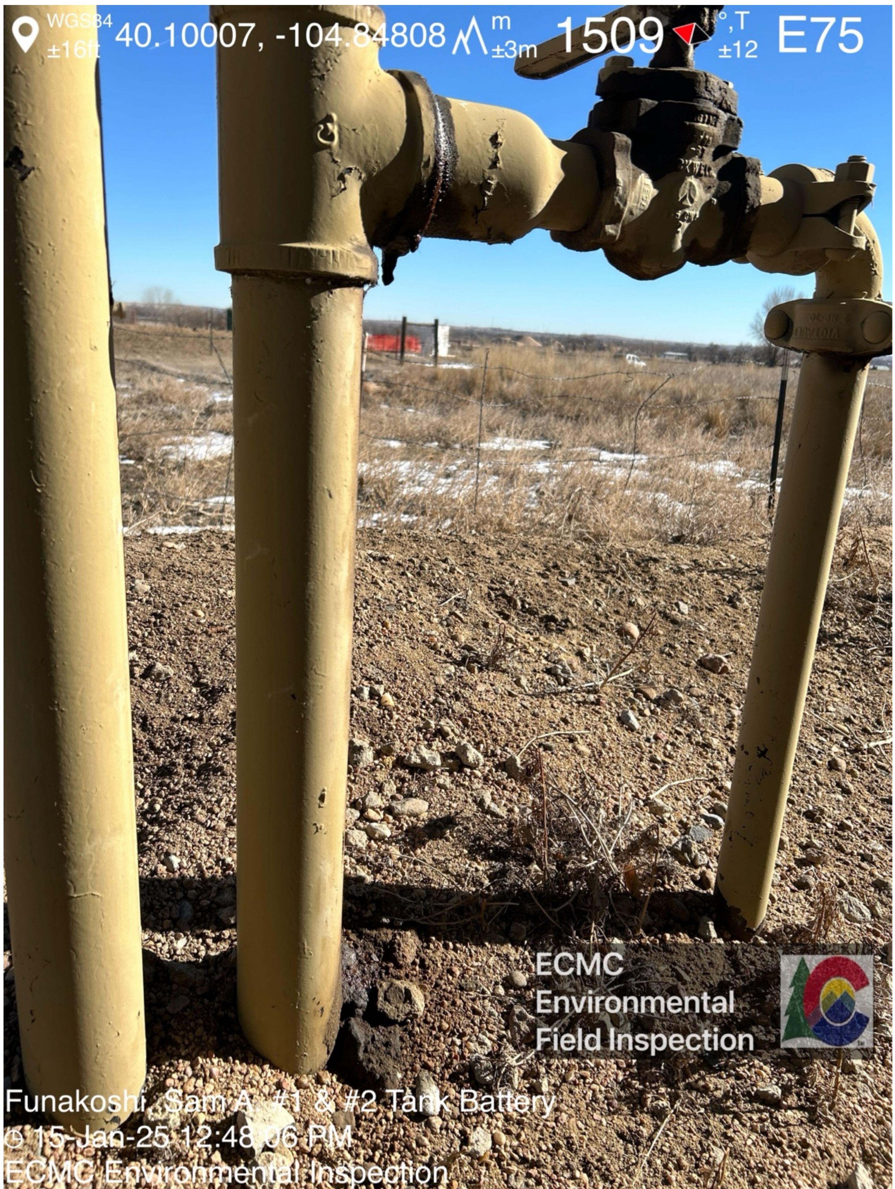
Petroleum hydrocarbon staining and odor observed on and beneath pipe manifold valve.
