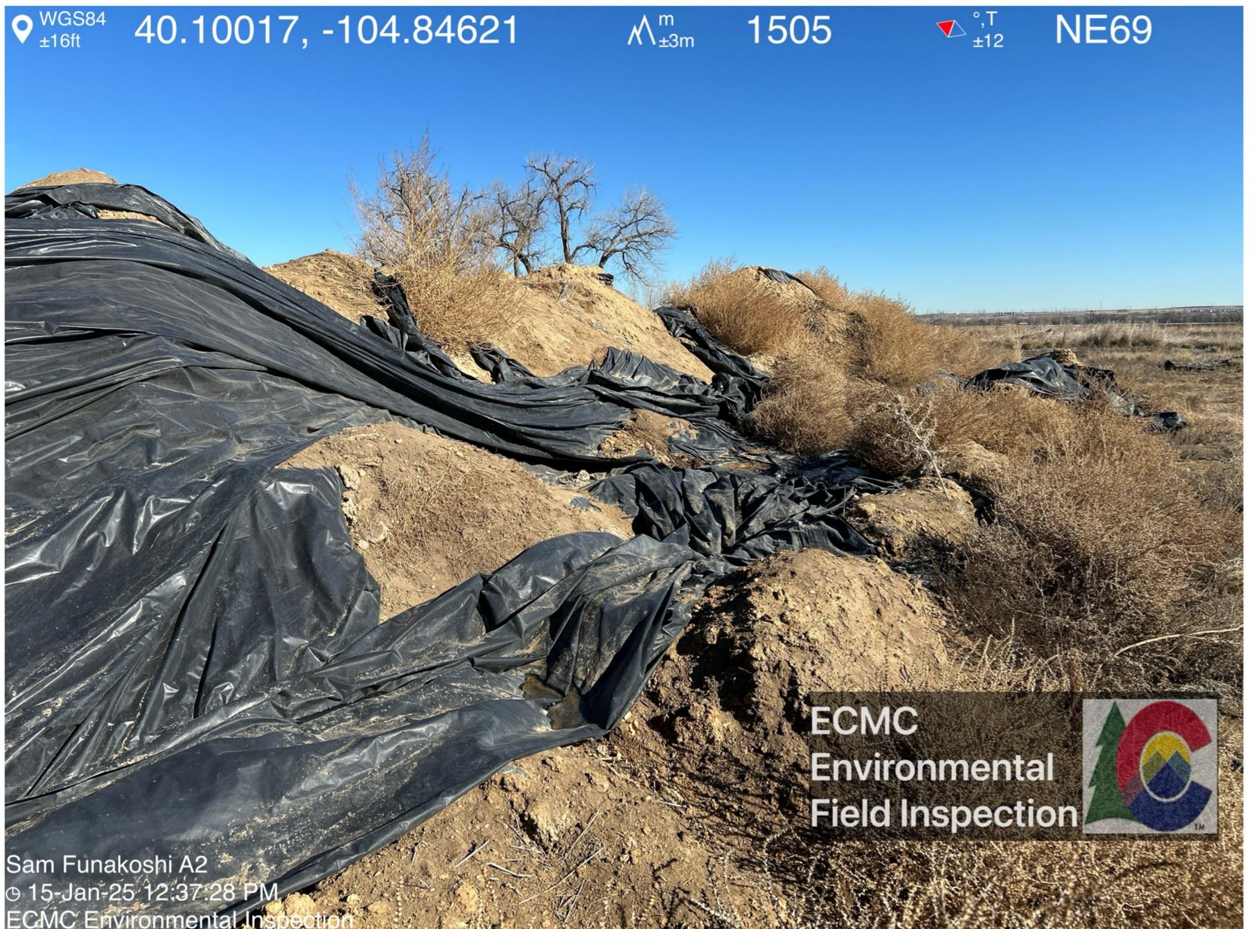
E&P waste has spilled outside of secondary containment. Weeds have grown on the stockpile.
