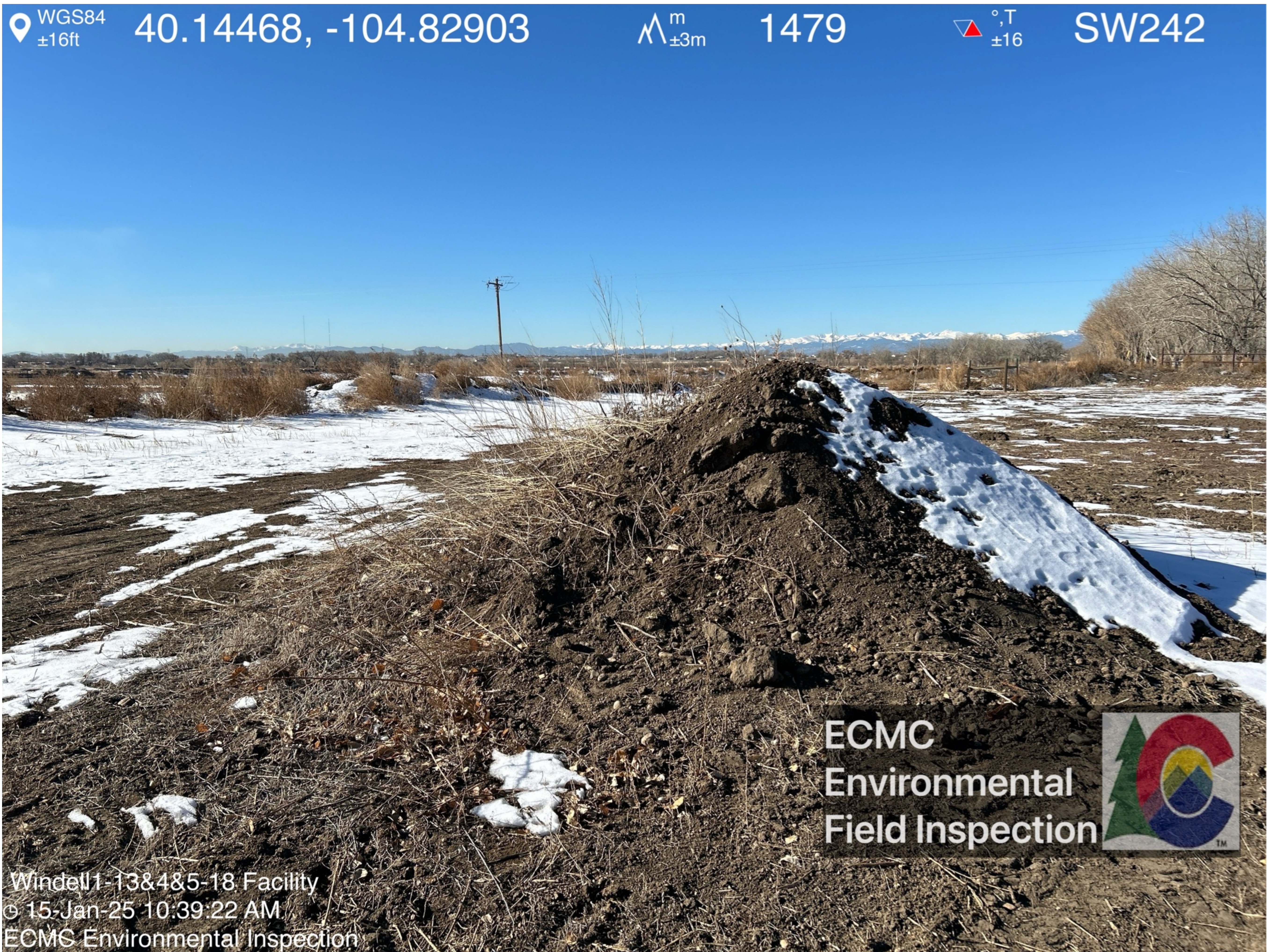
Soil stockpiled on location with inadequate BMPs.
