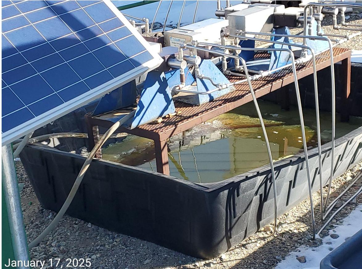
**Photo 3:** Fluids from the methanol pumps appears to have spilled into containment. Wildlife protection BMPs missing from containment measures.
