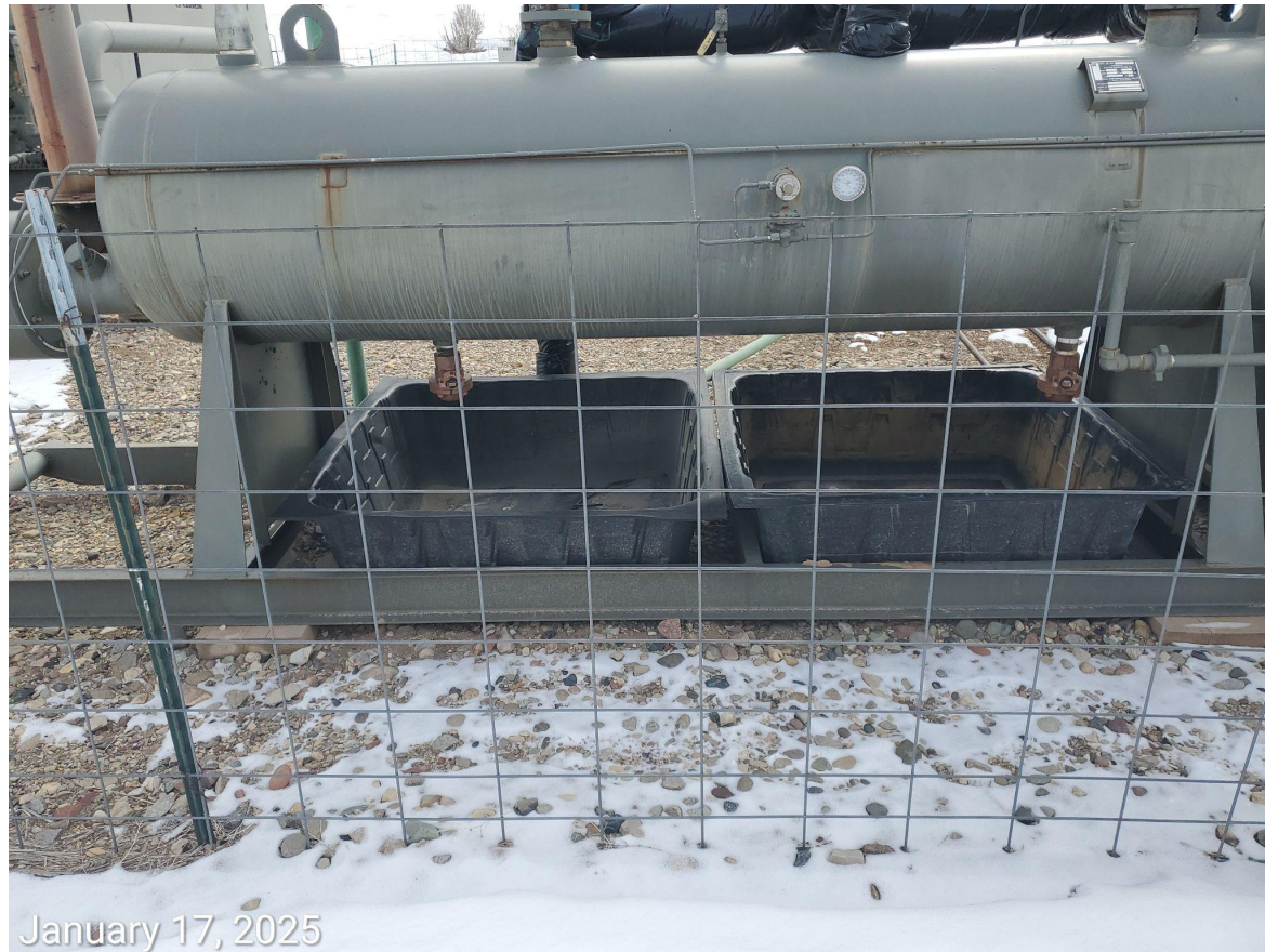
Photo 9: Wildlife protection measures missing from containment BMPs
