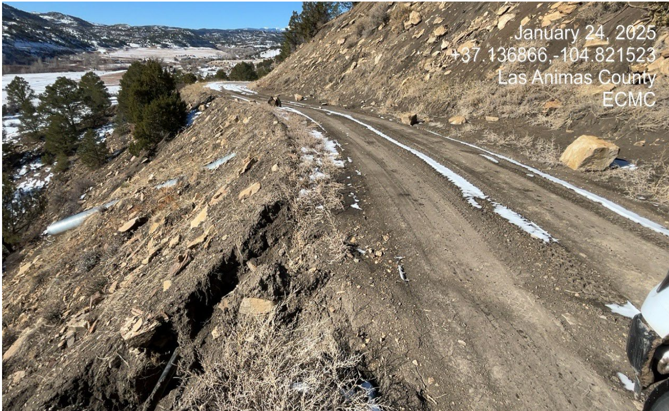
Photo 2. Facing southwest along the access road. The culvert is filled in with sediment at this area.
