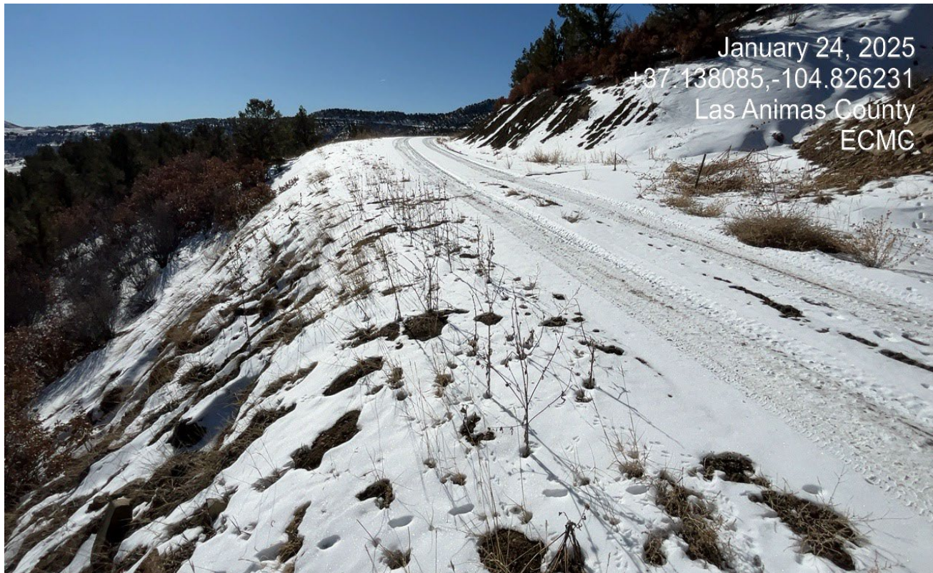
Photo 3. Facing southwest along the access road. It appears the culvert may be filled in and stormwater causing erosion along the road side at this area.
