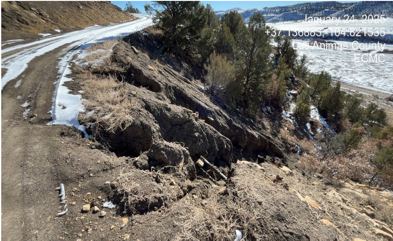
Photo 1. There is erosion occurring along the access road which needs to be repaired and stabilized..
