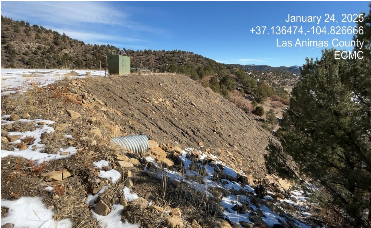
Photo 5. Facing east toward the fill slope. There are signs of erosion along the fill slope.
