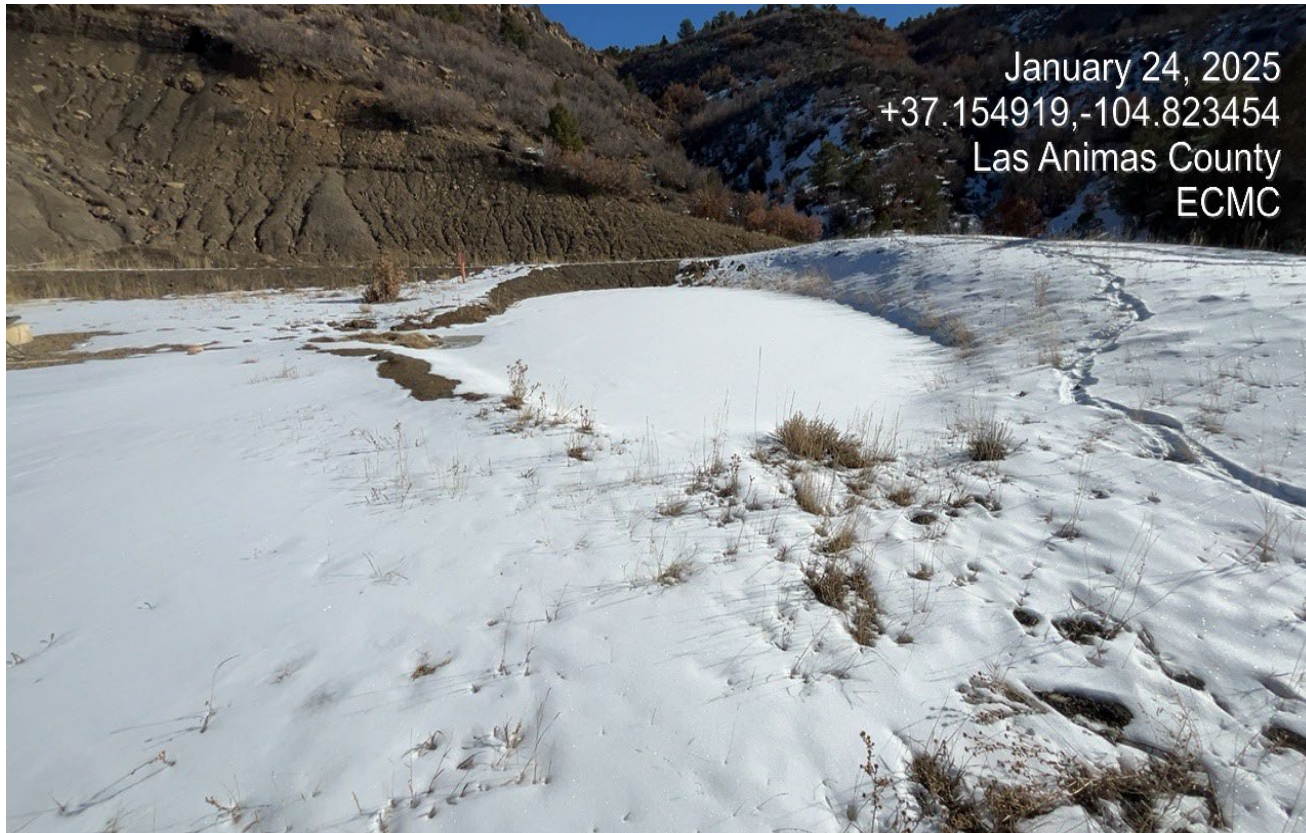
Photo 3. The pit at the south side of the location was nearing freeboard.
