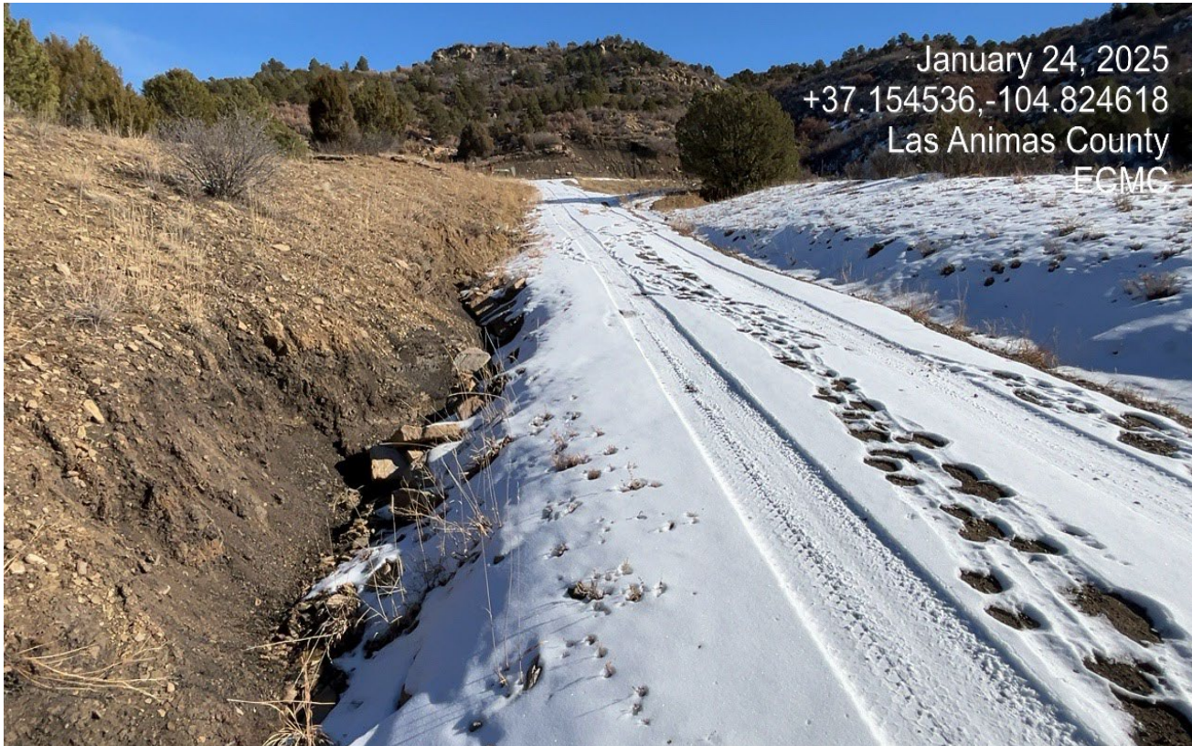
Photo 1. Facing northeast along the access road. Erosion occurred along the road side and rock check dams have been displaced.
