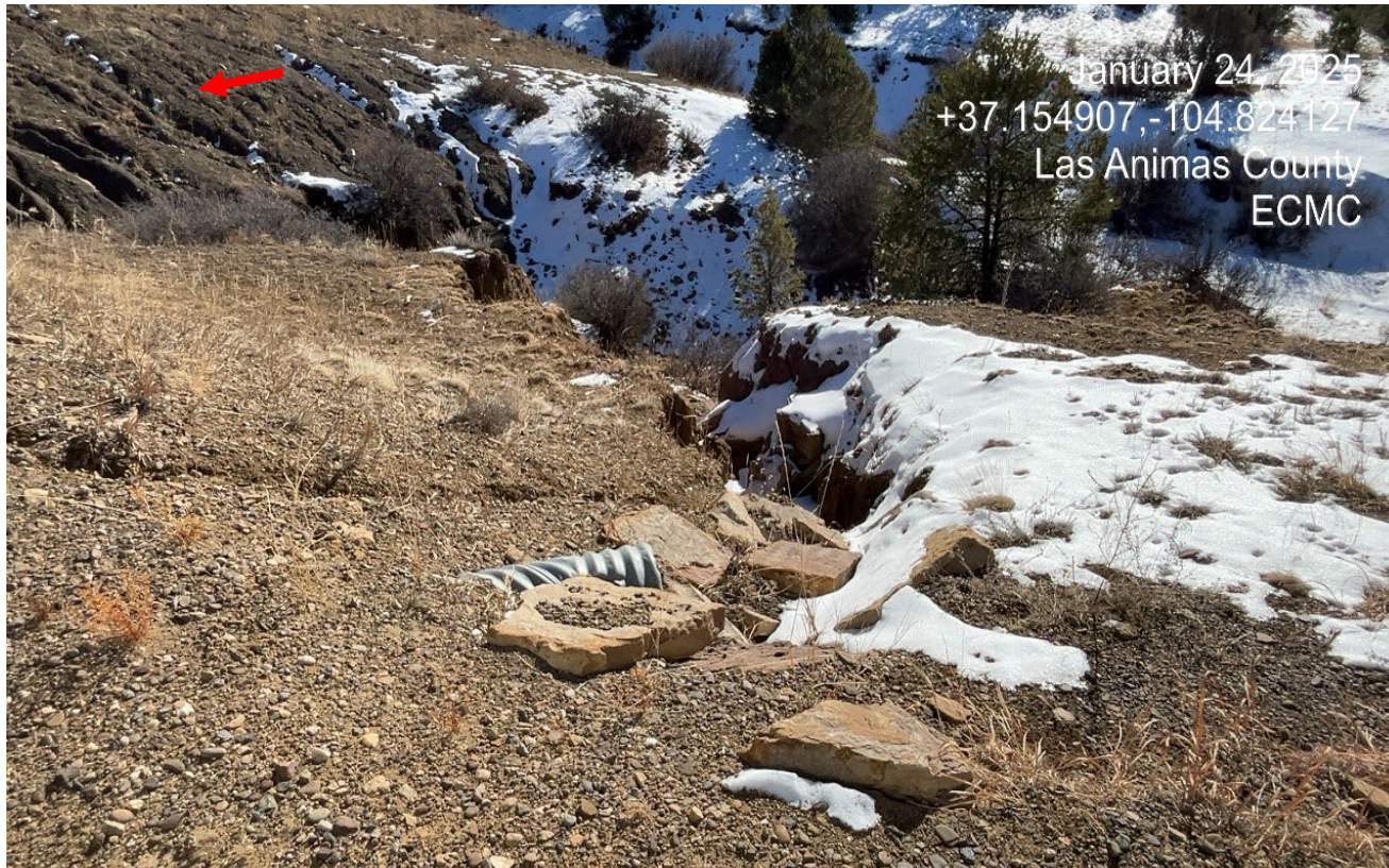
Photo 2. There is erosion at this culvert outlet and along the fill slope of the location shown at red arrow..
