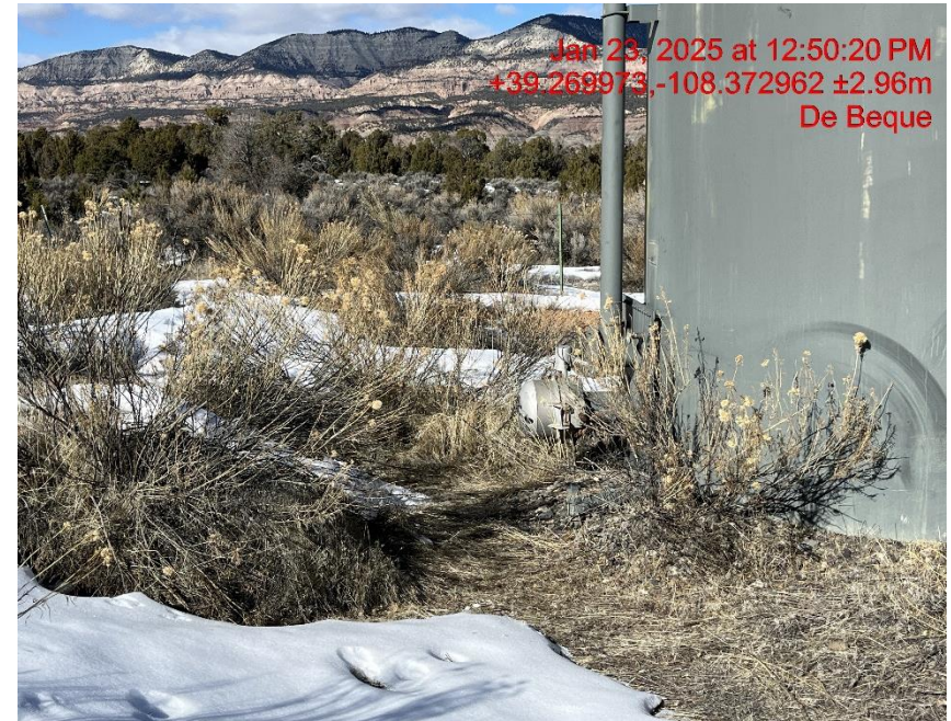
Photo # 3269 Weeds/undesirable plant species near production equipment causing a fire hazard
