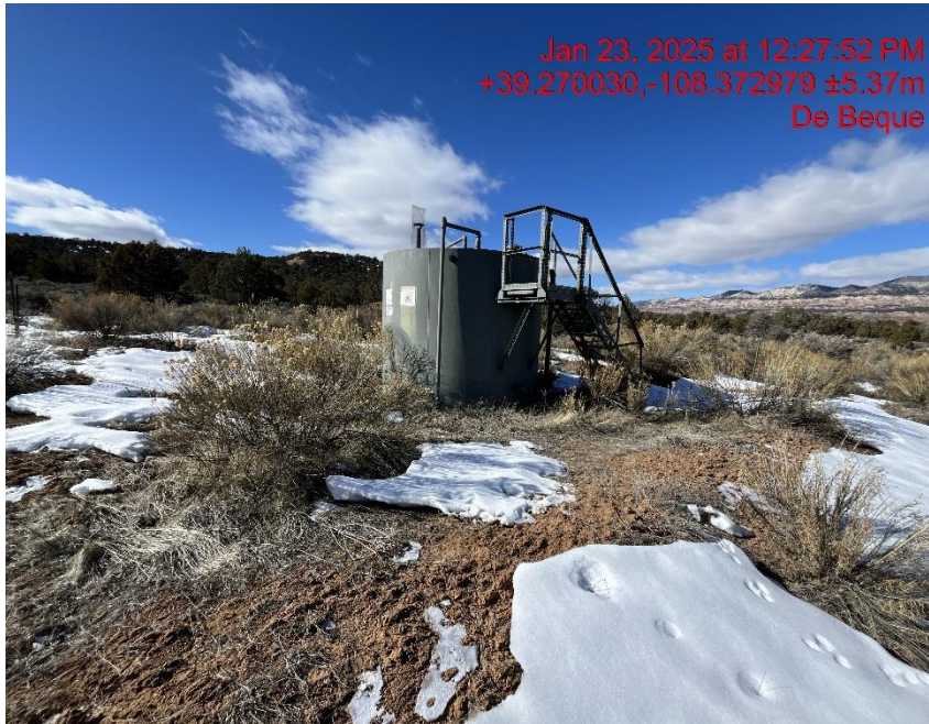
Photo # 3254 Secondary containment is insufficient/does not comply with CECMC rules. Additionally weeds/undesirable plant species inside secondary containment have compromised the containment
