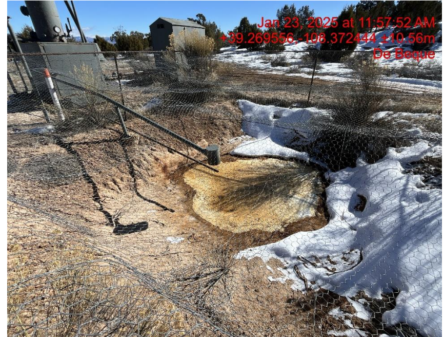
Photo #3237 Unlined Pit #1 appears to have condensate in it with weeds/undesirable plant species
