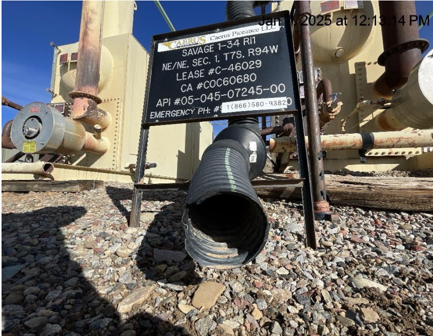
Photo # 7207 From audit 708905436 conducted on 01/07/2025 Flowline heating insulation open ended/wildlife hazard/available for entry by wildlife
