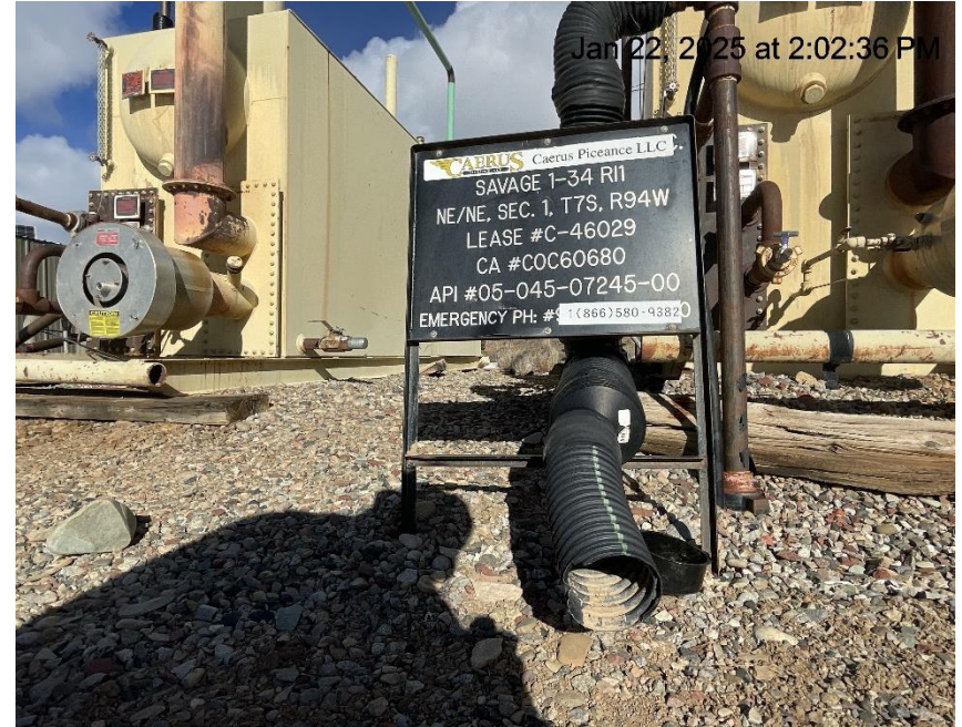
Photo # 753 Flowline heating insulation open ended /wildlife hazard/available for entry by wildlife
