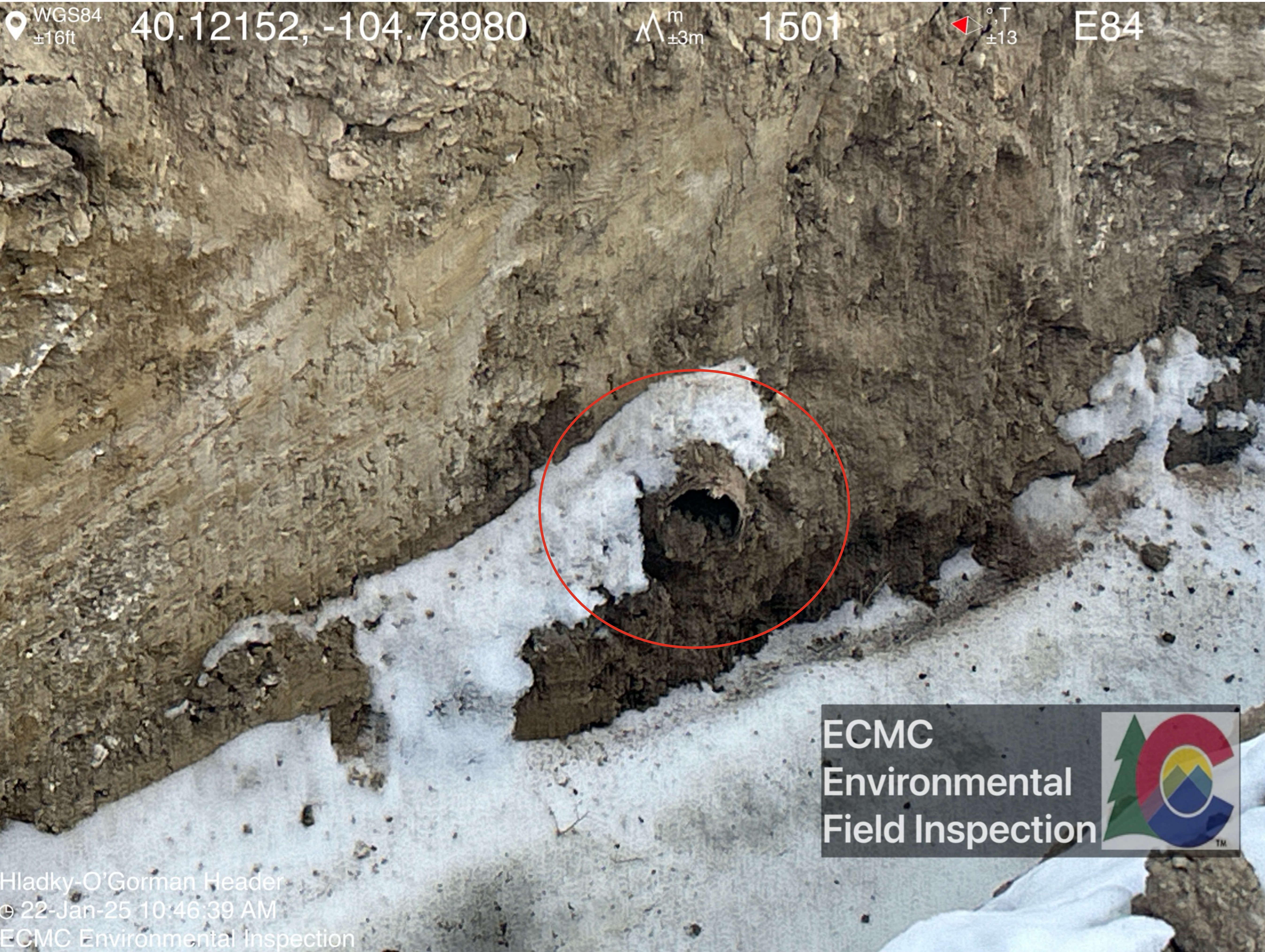
Severed pipe visible within trench.
