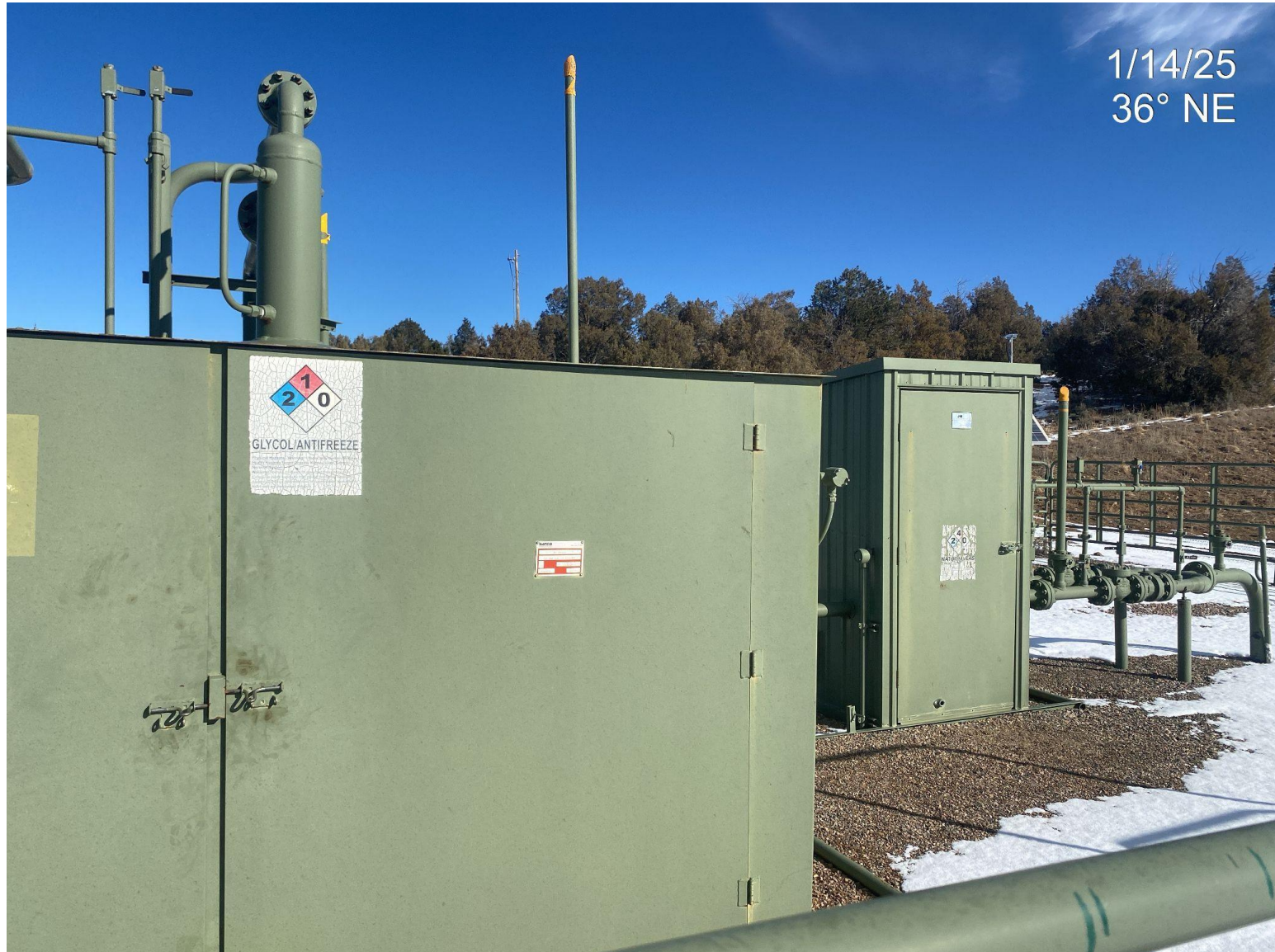
Photo 3. Labels at separator are deteriorating, future maintenance is advised.
