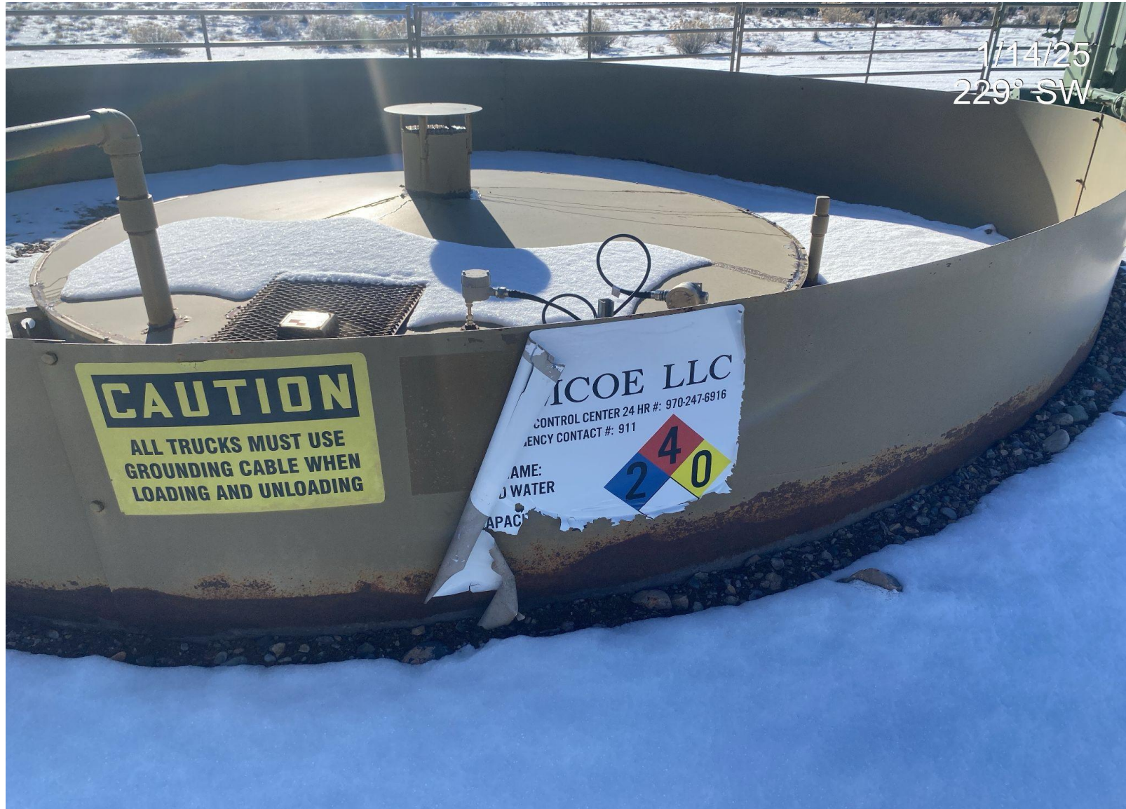
Photo 3. Produced water tank label has deteriorated and no longer legible.
