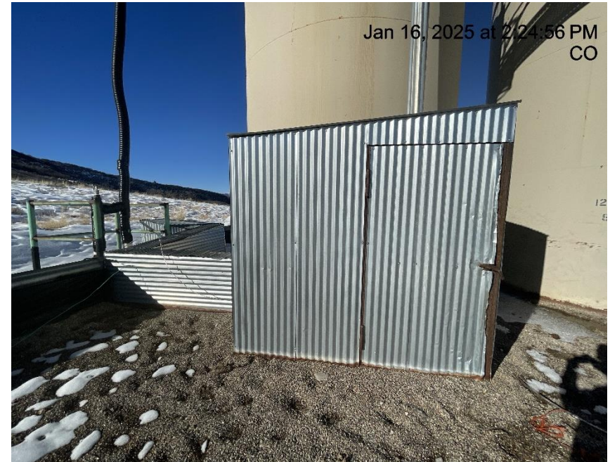
Photo # 9815 Shed inside secondary containment that has a catalytic heater inside
