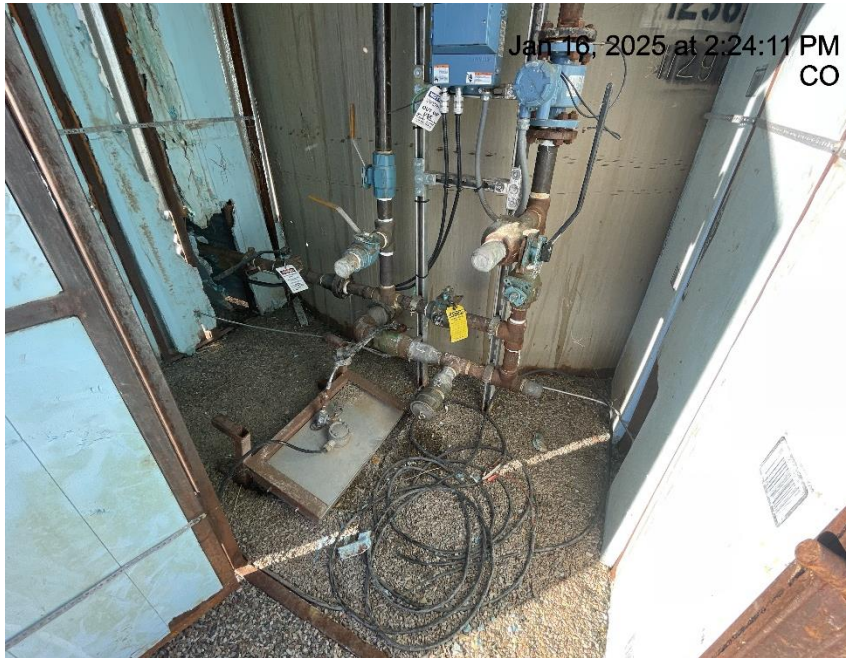
Photo # 9816 Catalytic heater inside secondary containment /fire & safety hazard
