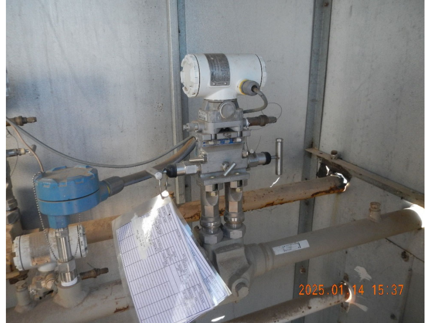
6. Gas meter inside meter shed.
