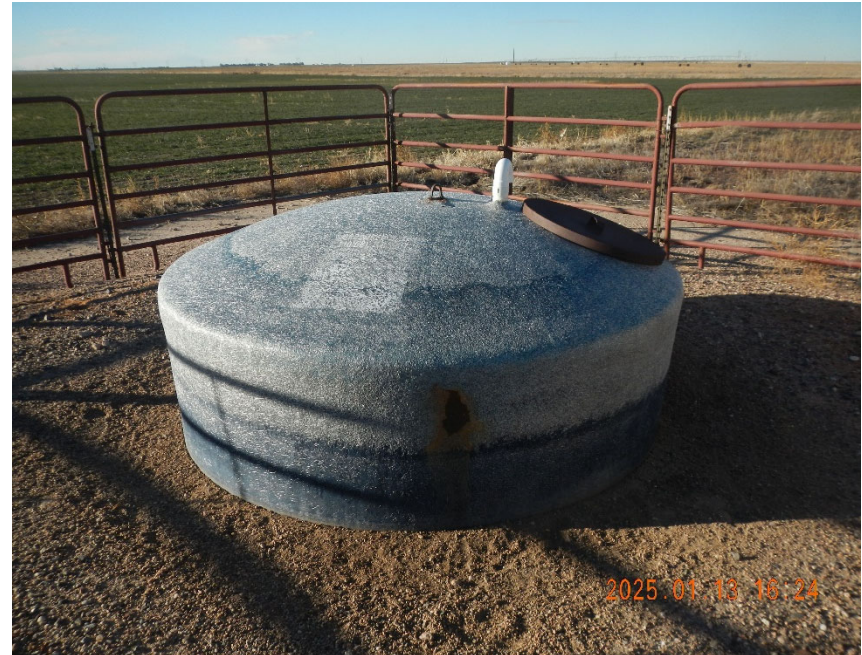
6. Produced water tank at gathering location. No sign or readable labels on tank.
