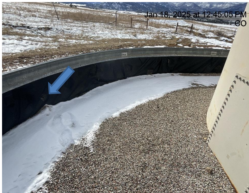
Photo # 237 Hole in liner/liner needs maintenance
