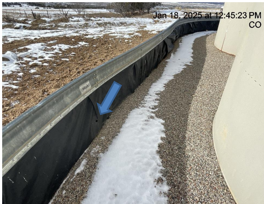
Photo # 239 Hole in liner/liner needs maintenance
