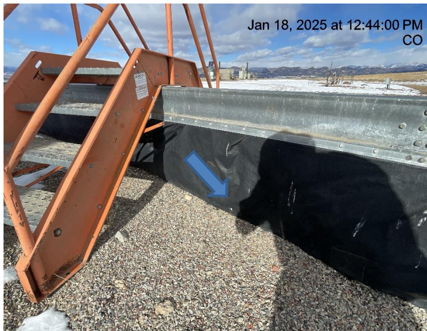
Photo # 235 Hole in liner/liner needs maintenance
