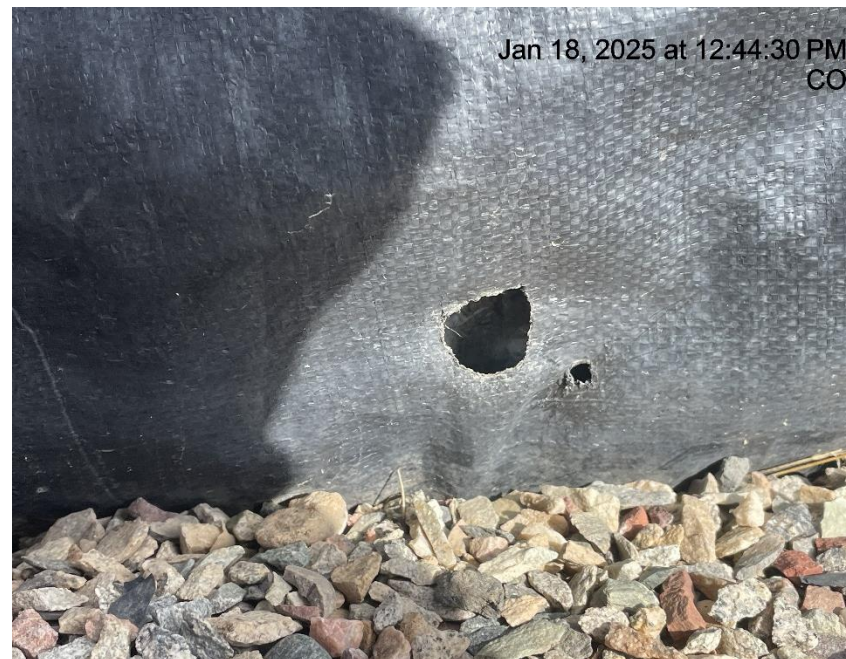
Photo # 236 Hole in liner/liner needs maintenance
