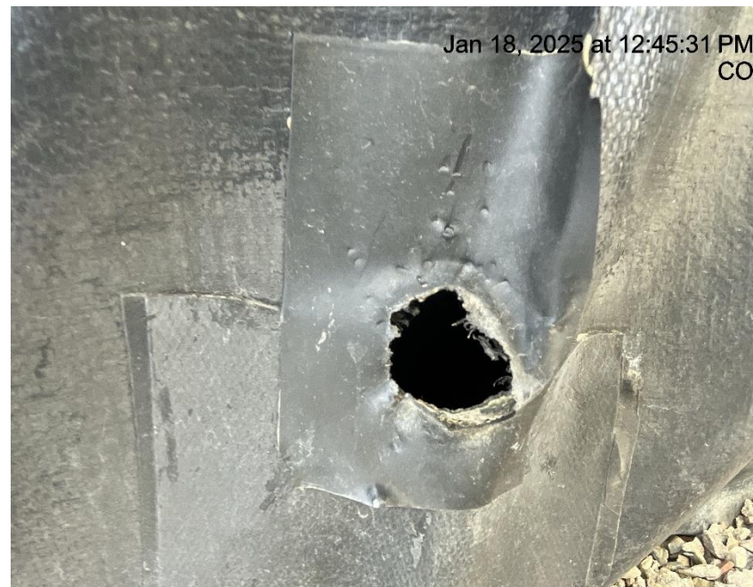
Photo # 240 Hole in liner/liner needs maintenance
