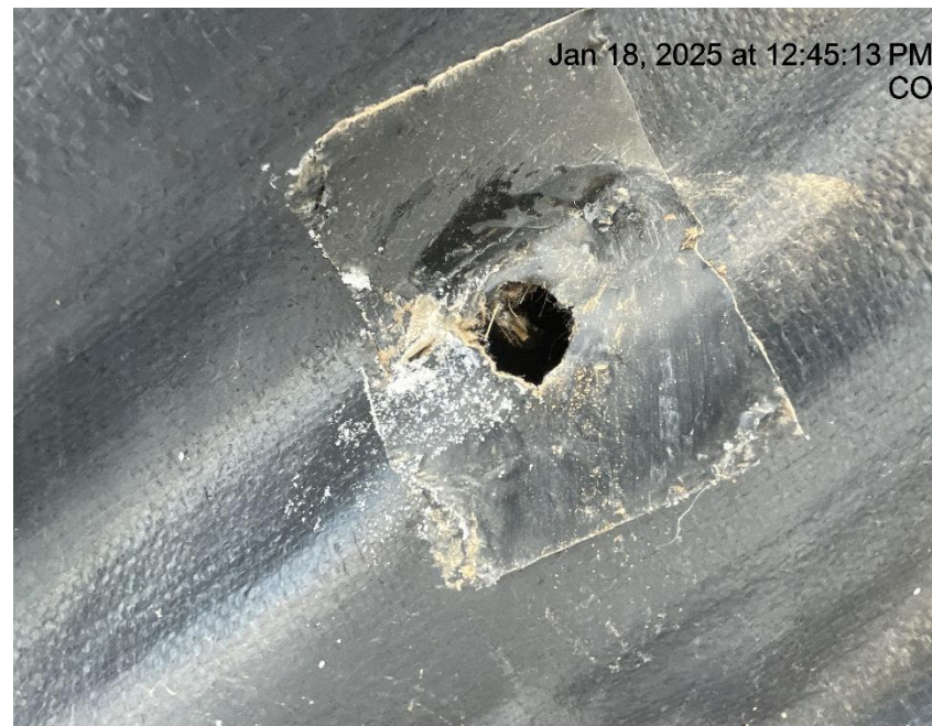
Photo # 238 Hole in liner/liner needs maintenance
