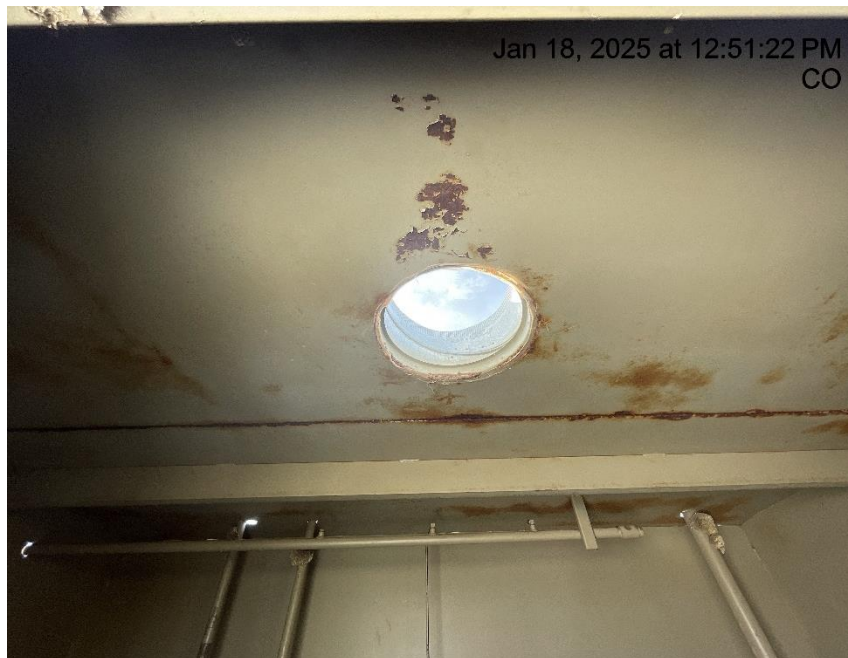
Photo # 241 Hole in separator/wildlife hazard/available for entry by wildlife
