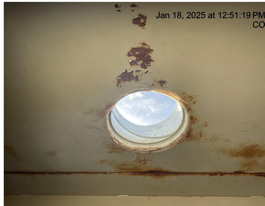
Photo # 242 Hole in separator/wildlife hazard/available for entry by wildlife
