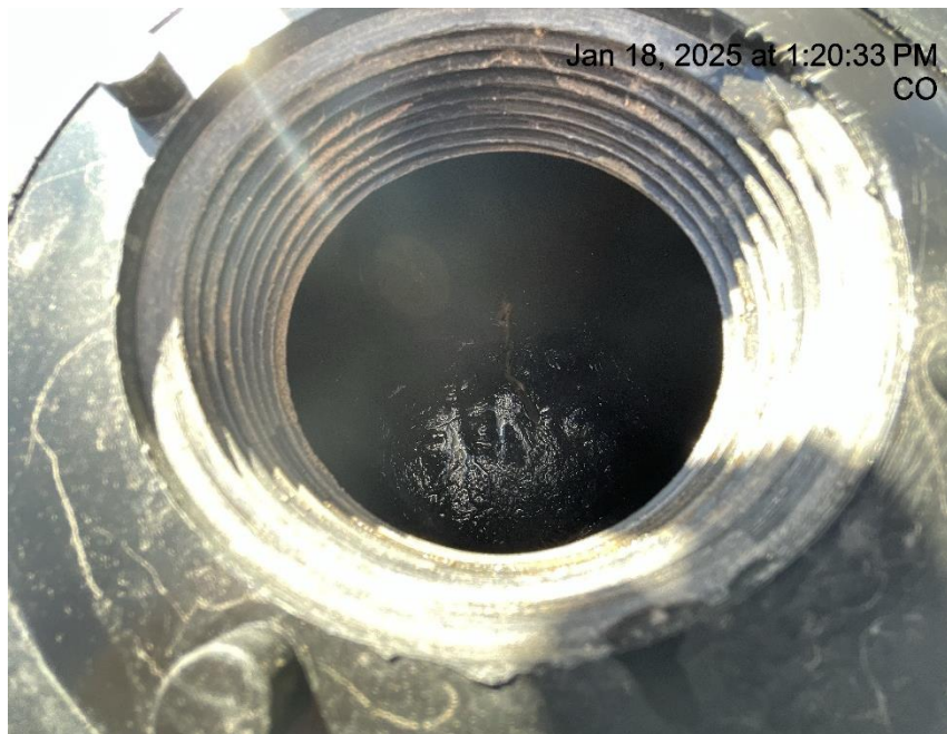
Photo # 360 Failure to maintain chemical BMP – Chemical tank containment approximately 2/3 full of fluid/BMP insufficient to contain possible spill
