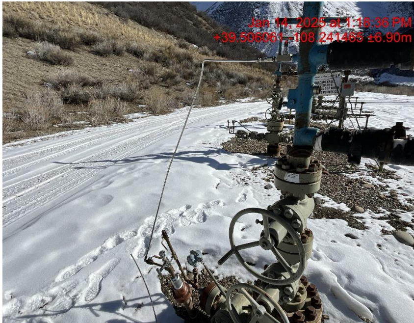
Photo # 2746 Bradenhead line tied into flowline/no FORM 4 SUNDRY/not in compliance with CECMC rules
