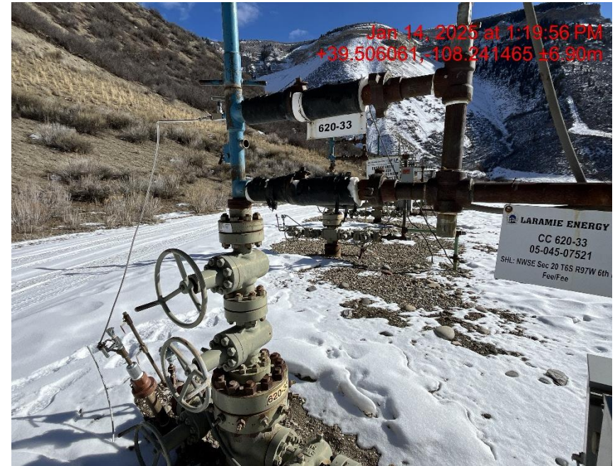
Photo # 2748 Bradenhead line tied into flowline/no FORM 4 SUNDRY/not in compliance with CECMC rules
