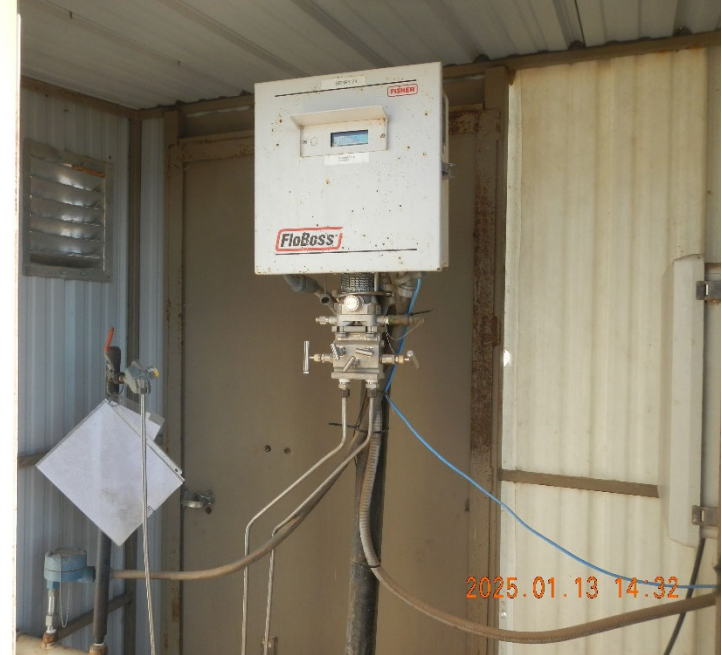
6. Gas meter inside meter shed.
