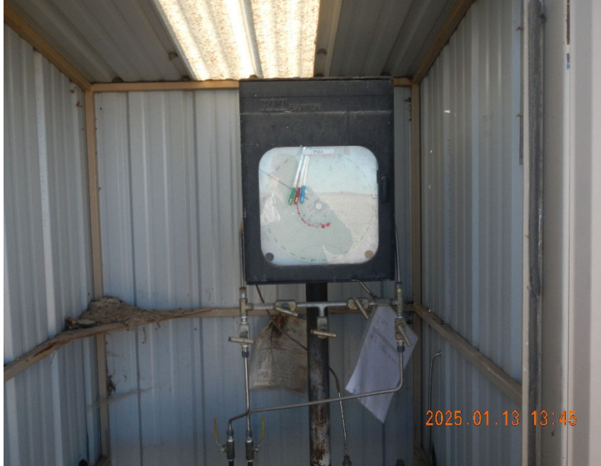
5. Gas meter inside meter shed.
