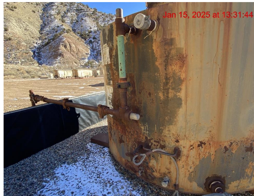
Corrosion on Storage Tank – Photo #05991
