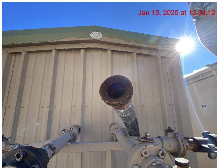
Open-Ended Line Near Gas Meters – Photo #05995
