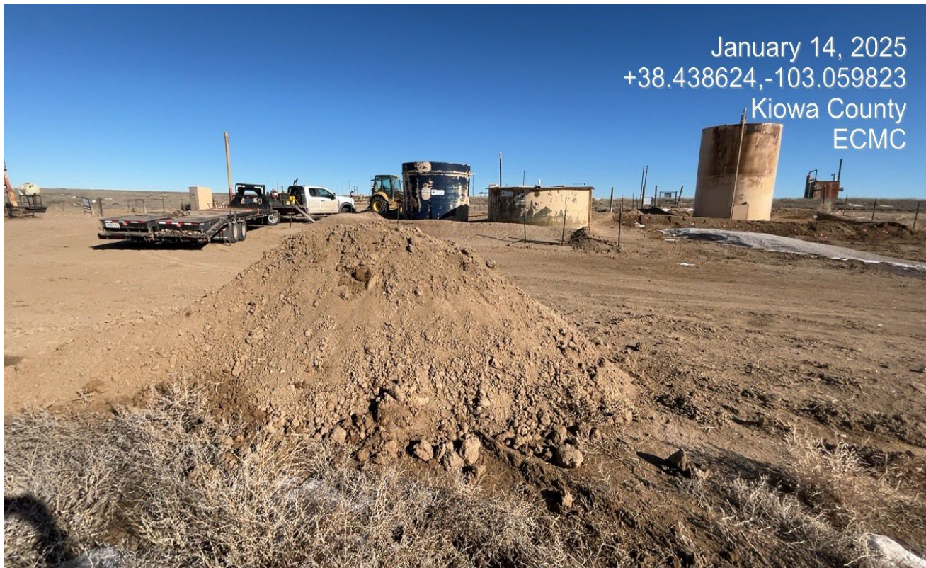
Photo 5. South side of the location facing north. There is a pile of material which has hydrocarbon impacts stored with no liner or containment. This appears to be part of the impacted berm material.
