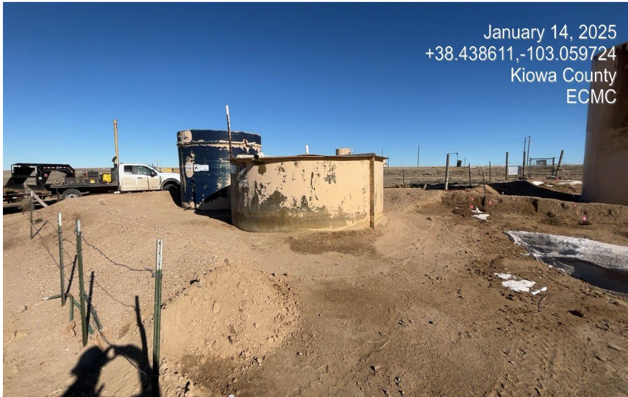
Photo 6. Facing toward the two fiberglass tanks. There is no secondary containment around the tanks which should be empty and not in use without containment.
