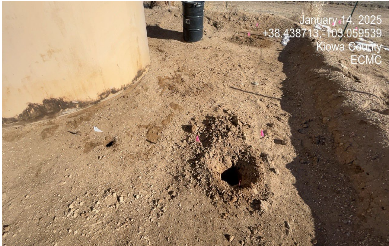
Photo 8. Facing adjacent to the tank. There are still hydrocarbon impacted soils around the entire tank which have not been cleaned up.
