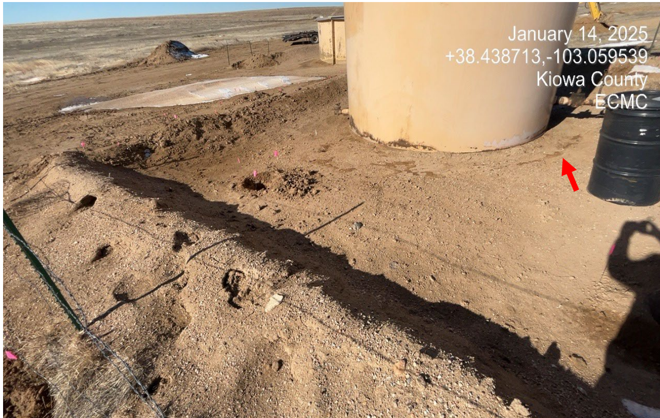
Photo 9. There are still impacted soils around the entire tank where spill had occurred. The tank will need to be removed to excavate and remove all of the impacted soils.
