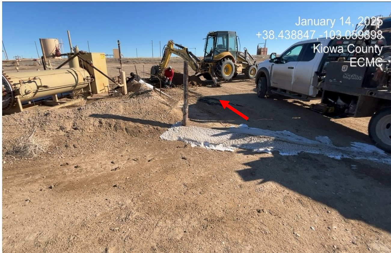
Photo 4. There were workers onsite repairing a leak along the flowline. There were oil stained soils at red arrow that will need to be cleaned up.
