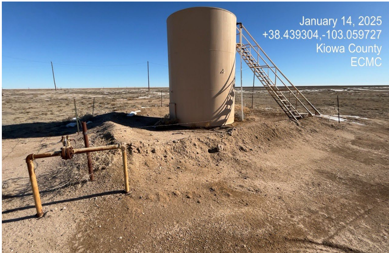
Photo 11. Facing at the north side of the location. The fence around the tank battery is inadequate to prevent livestock entry. The berm around the tank has been rebuilt.
