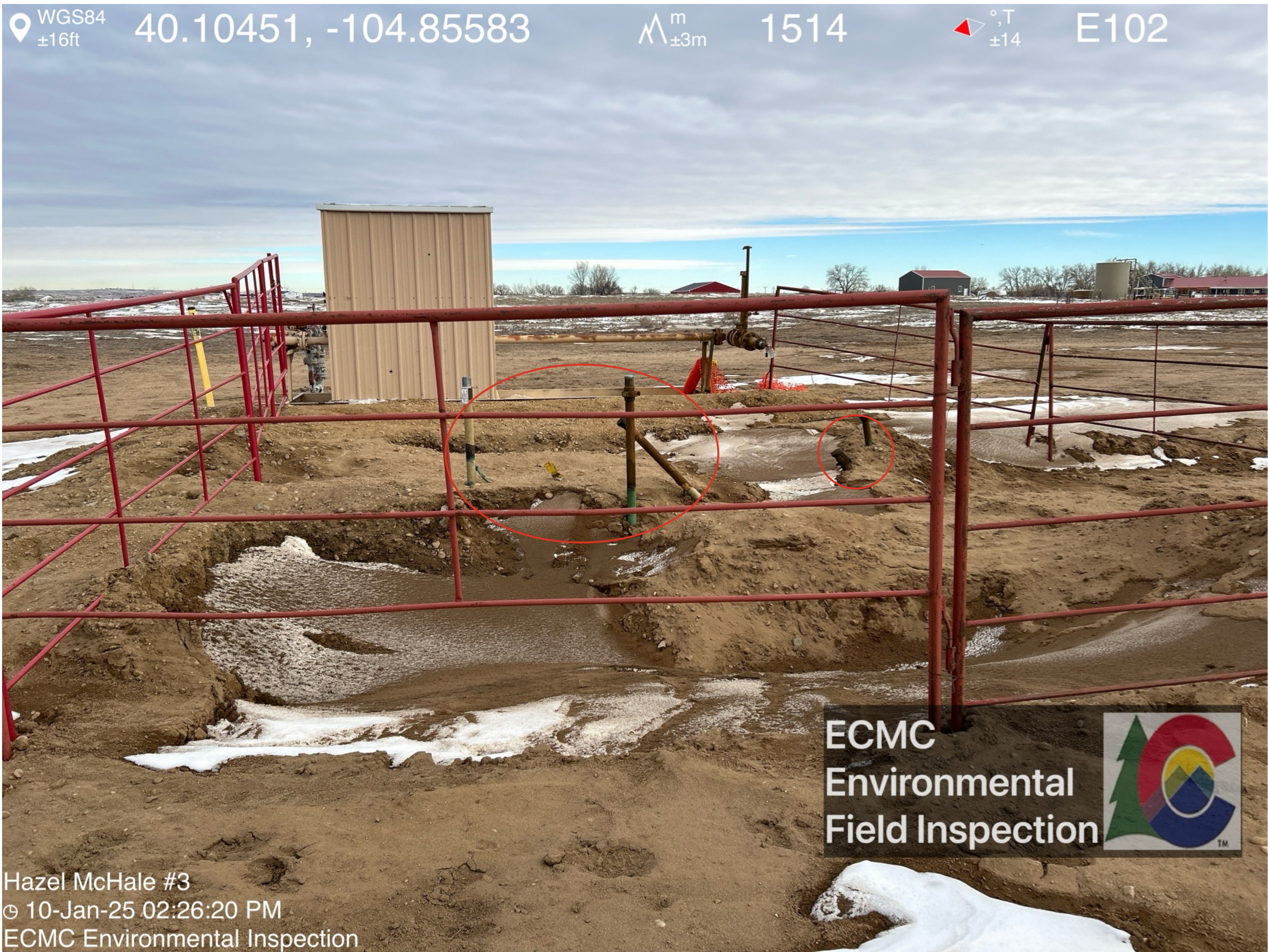
Multiple flowlines/flowline risers exposed within excavation.
