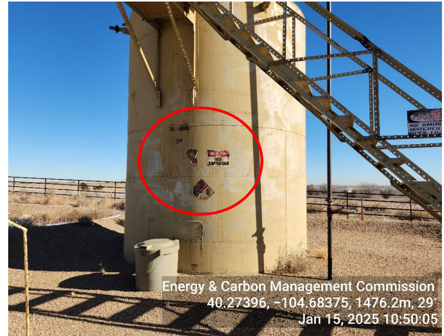
Photo 2: No capacity, contents displayed
