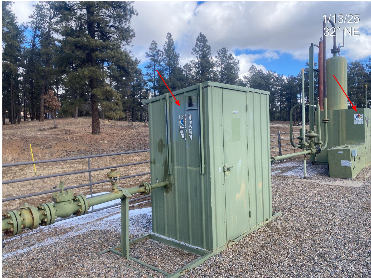
Photo 2. View of separator labels that have deteriorated and are no longer legible.
