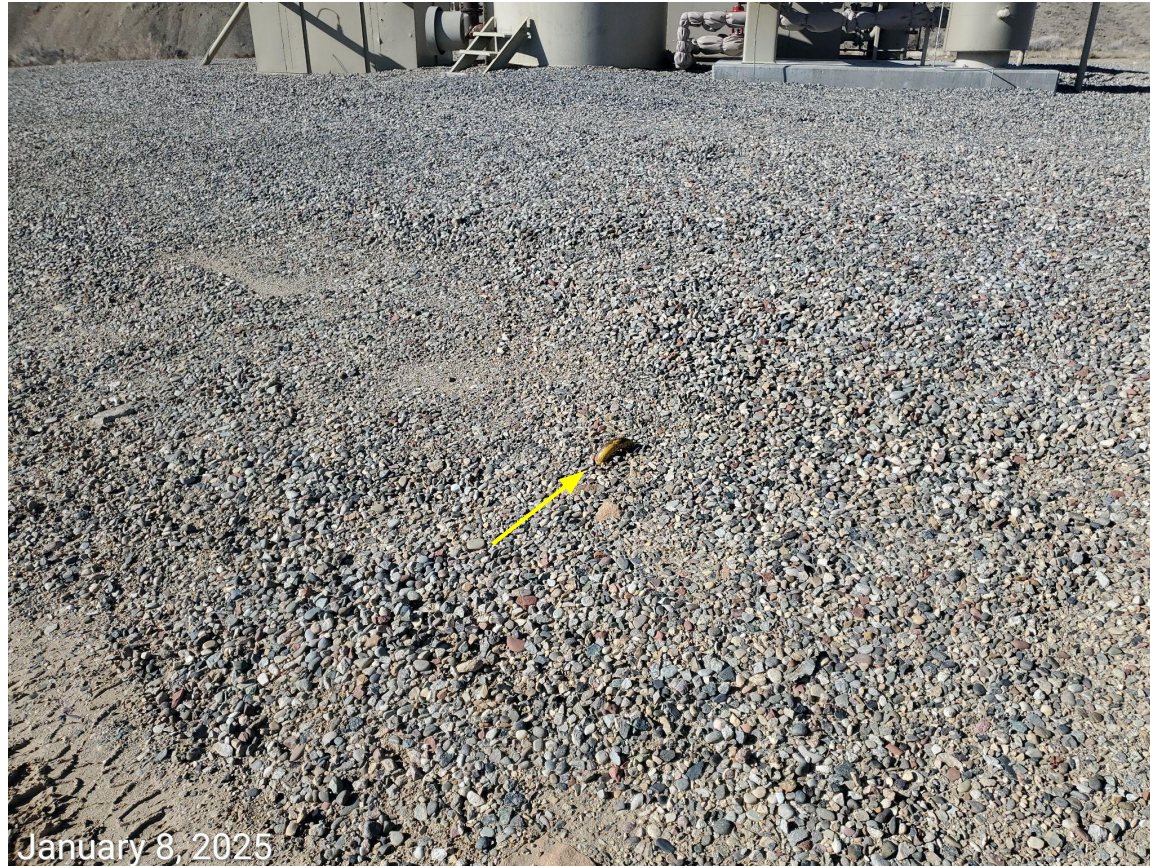
Photo 4: Photo example showing unmarked anchor (arrow) on the Location.
