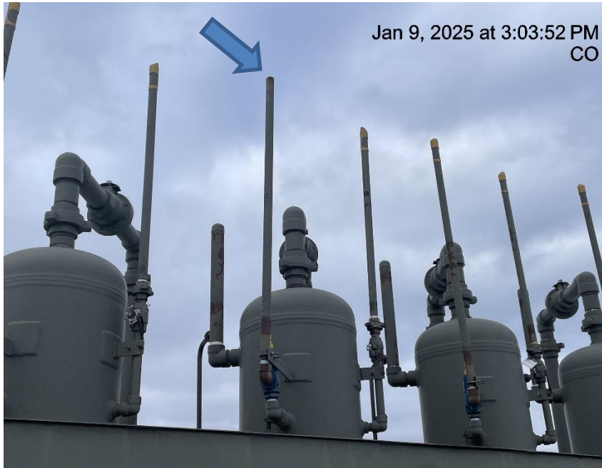
Photo # 8092 PRV vent line does not comply with CECMC pressure safety device rules
