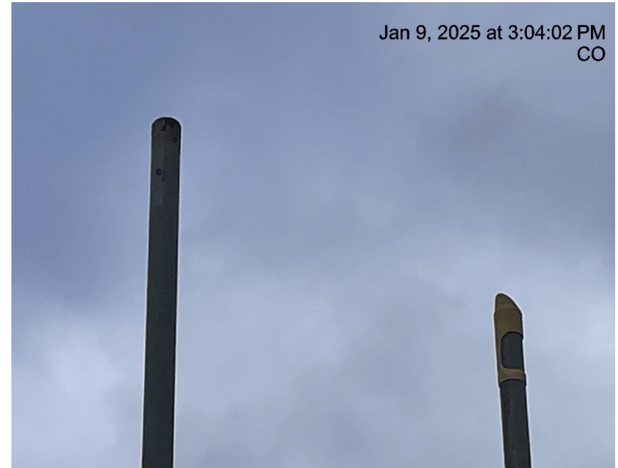
Photo # 8093 PRV vent line does not comply with CECMC pressure safety device rules
