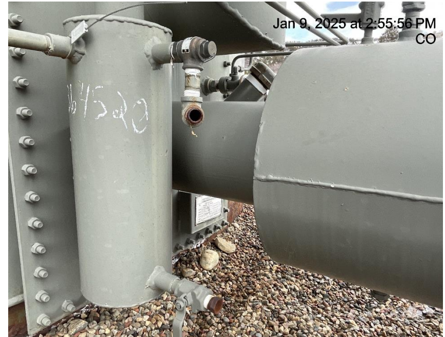
Photo # 8091 PRV vent line does not comply with CECMC pressure safety device rules
