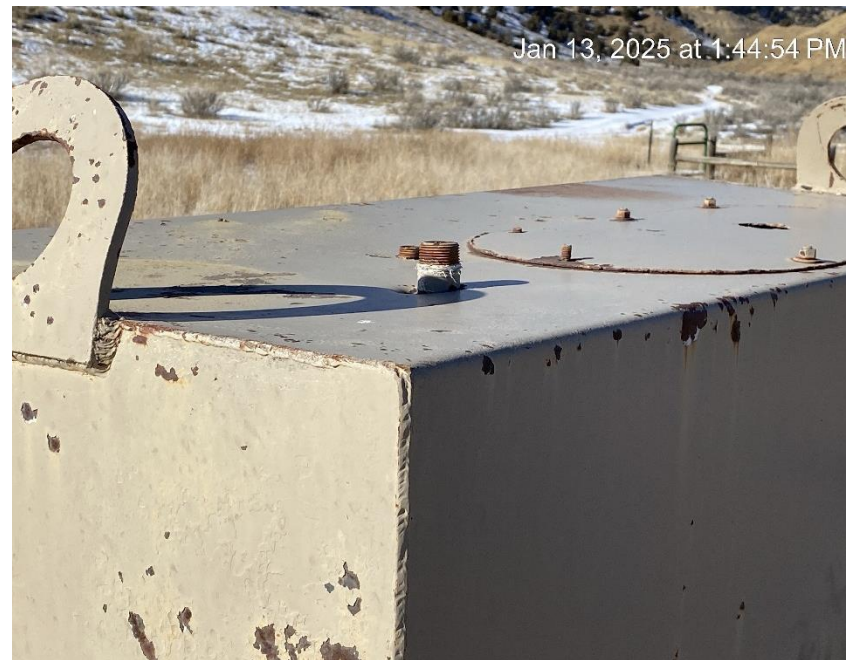
Unprotected vent risers
