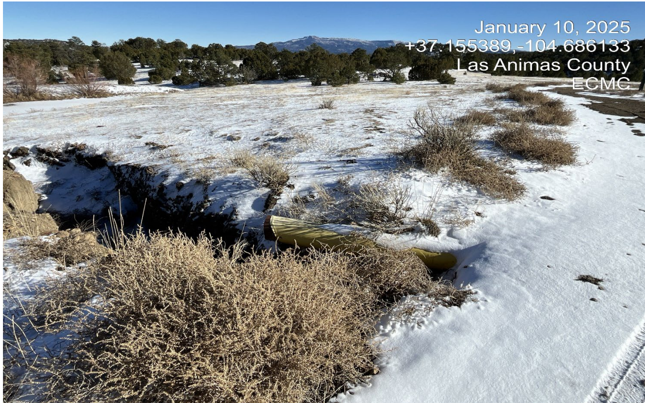
Photo 3. Facing east at the culvert outlet along the road. The culvert outlet has eroded and needs to be repaired and outlet protection installed.
