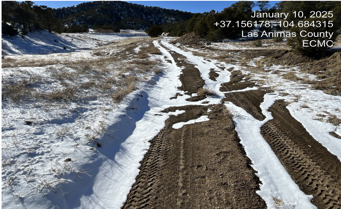
Photo 2. Facing west further along the access road. There is erosion along the road that needs to be repaired and stabilized.
