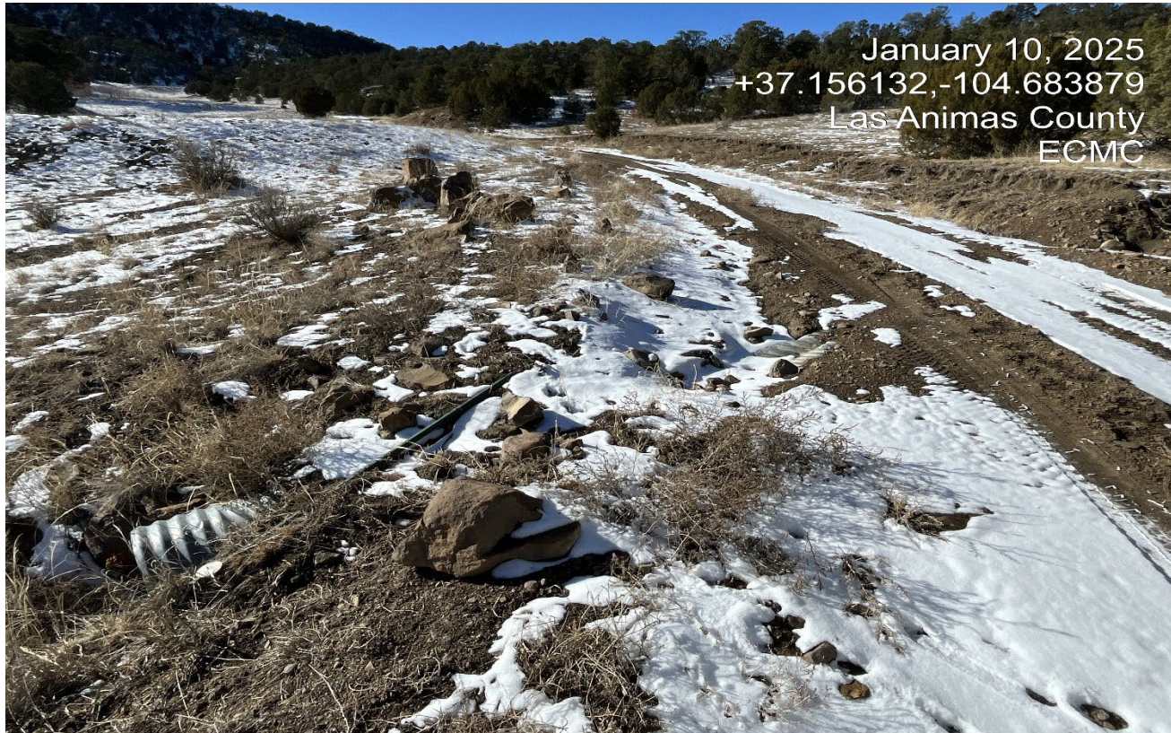
Photo 1. Facing west along the access road. There is erosion along the road that needs to be repaired and stabilized..
