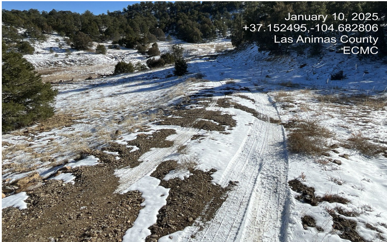
Photo 4. Facing southwest along the access road. There is erosion occurring across the road at this area.
