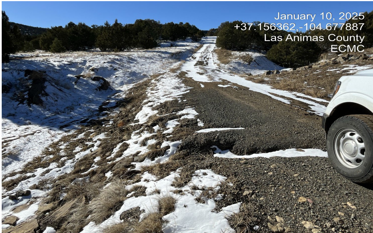
Photo 4. Facing southwest at the drainage crossing at the west side of the location. The culvert has filled in with sediment and stormwater has begun to erode the road.
