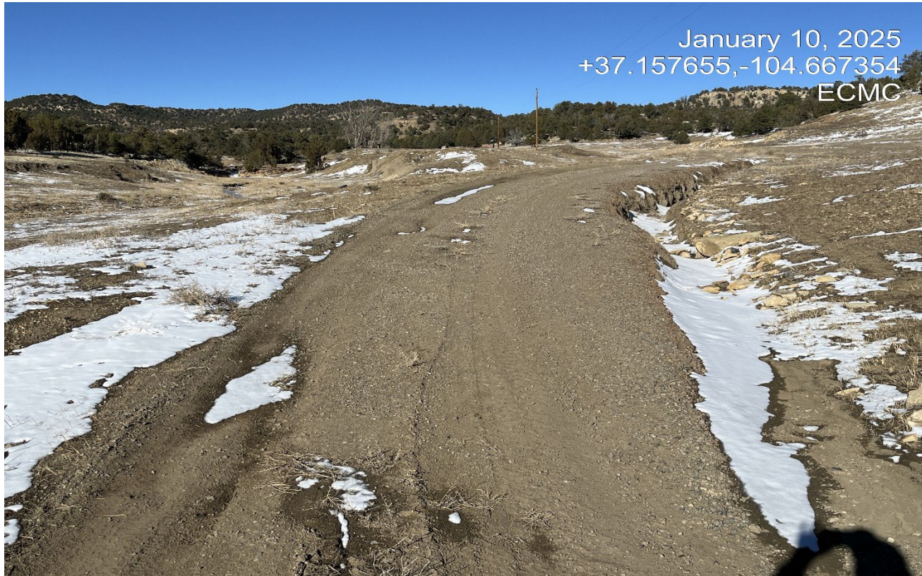
Photo 1. Facing northeast along the access road. There is erosion occurring along the roadside that will need to be repaired and stabilized.
