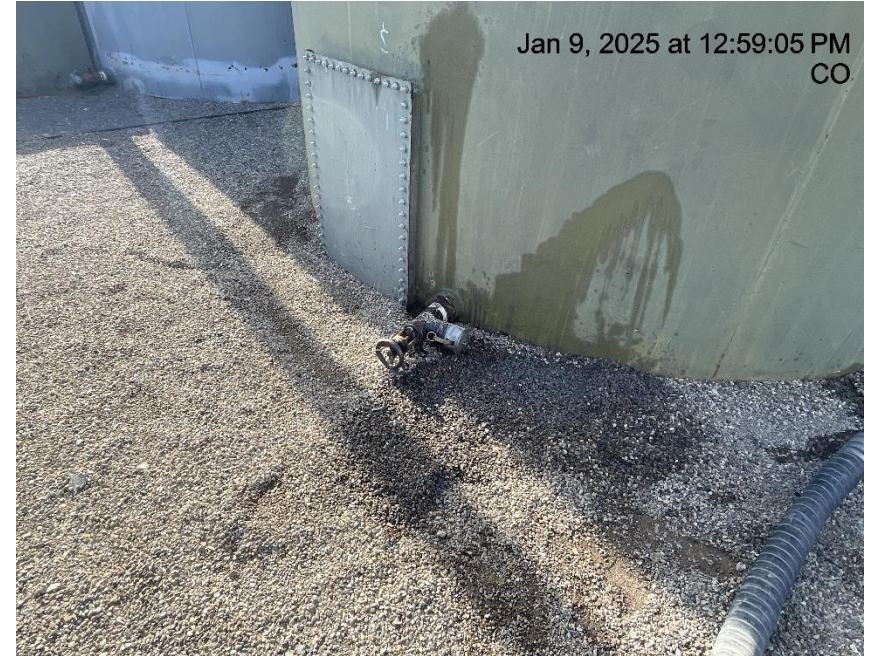
Photo # 7692 Staining in secondary containment
