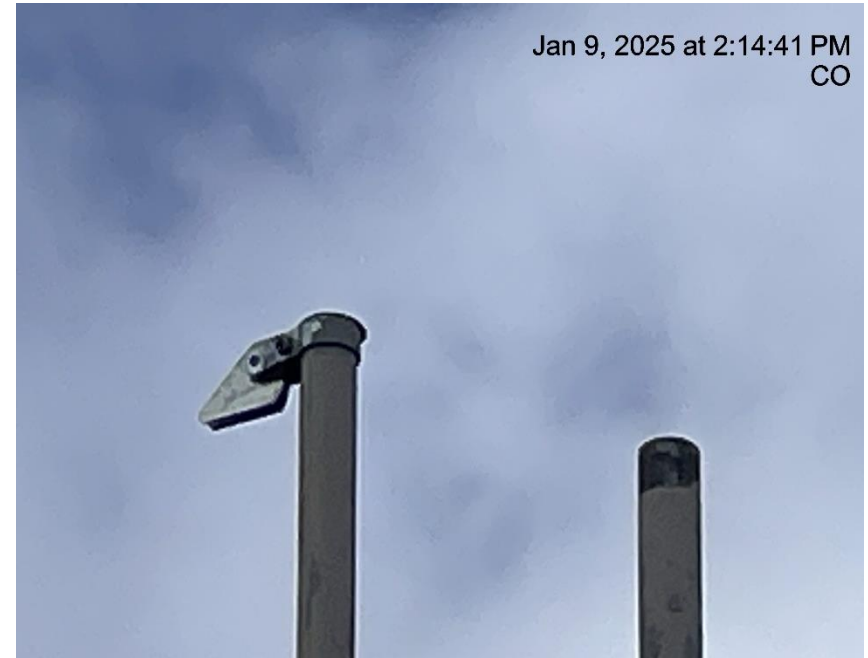
Photo # 7871 PRV vent line does not comply with CECMC pressure safety device rules
