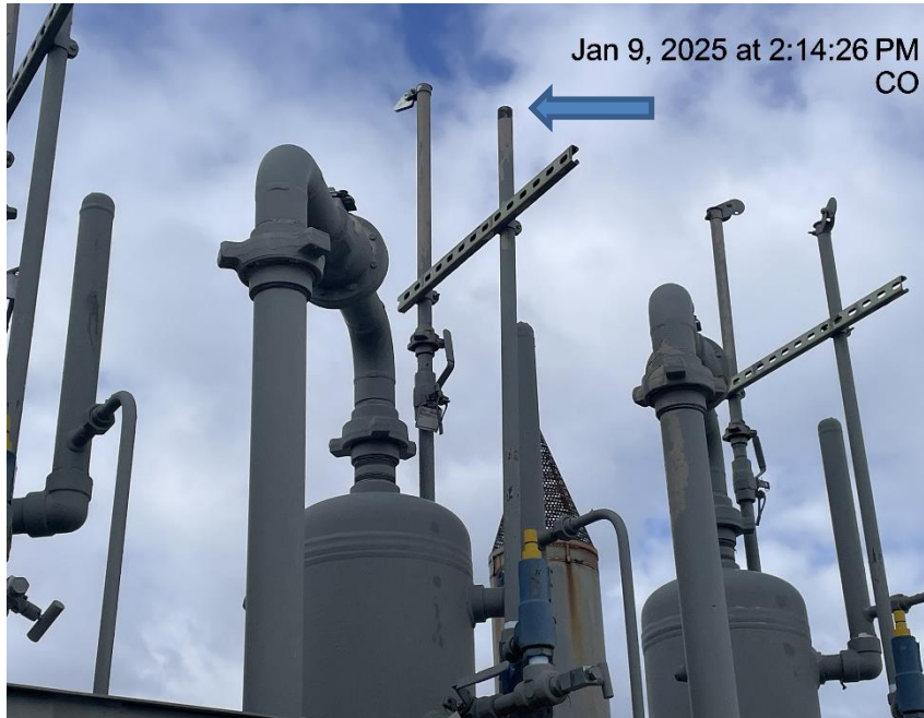
Photo # 7870 PRV vent line does not comply with CECMC pressure safety device rules
