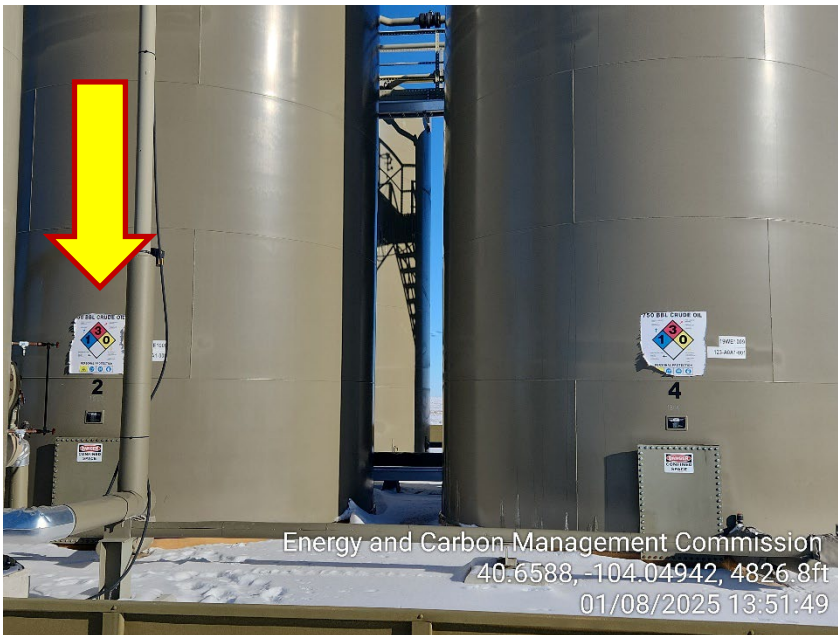
Photo 3 – Capacity Label is fading; replace soon
