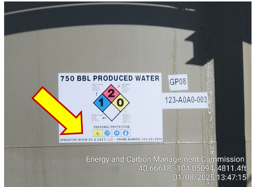
Photo 6 – 24-Hour Contact Name and Number are not current
