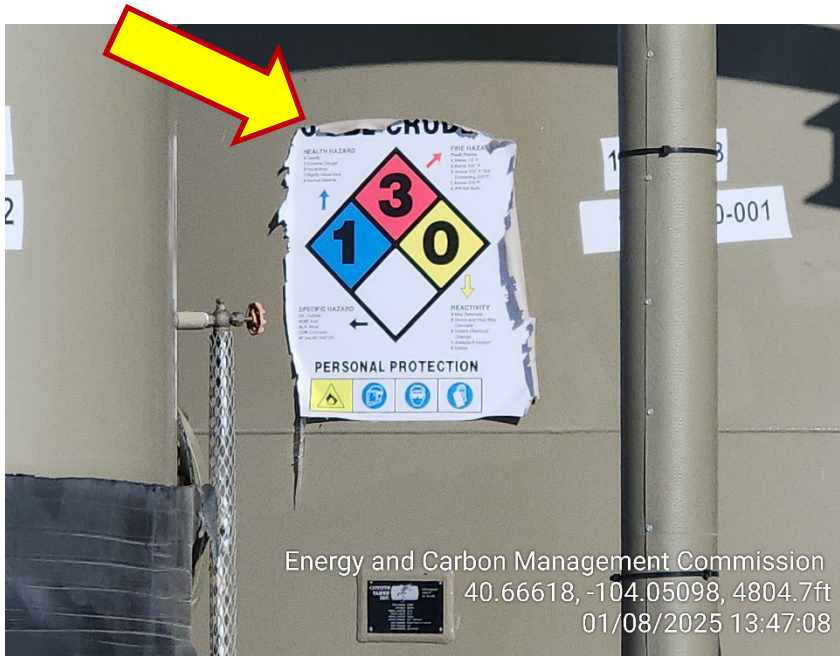
Photo 5 – Tank Label missing Content and Capacity Label
