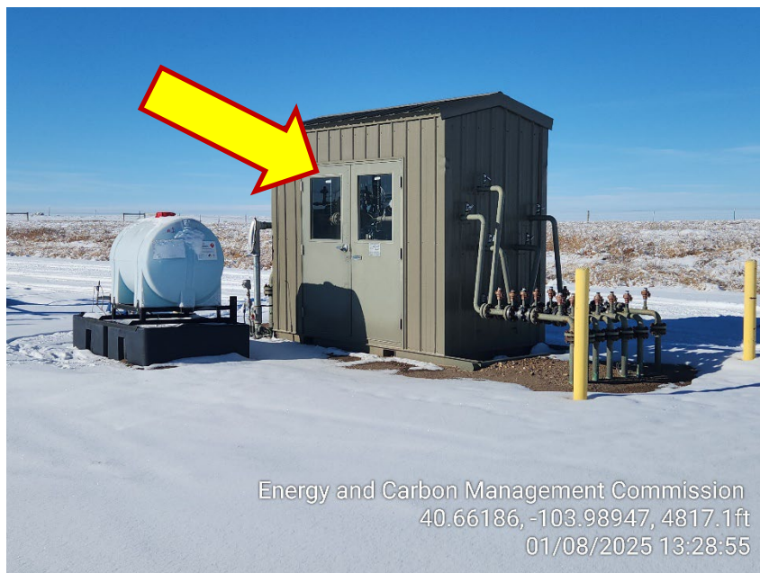
Photo 7 – Gas Lift Injection Meter House
