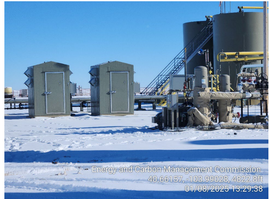
Photo 10 – VRU and Instrumental Air Unit
