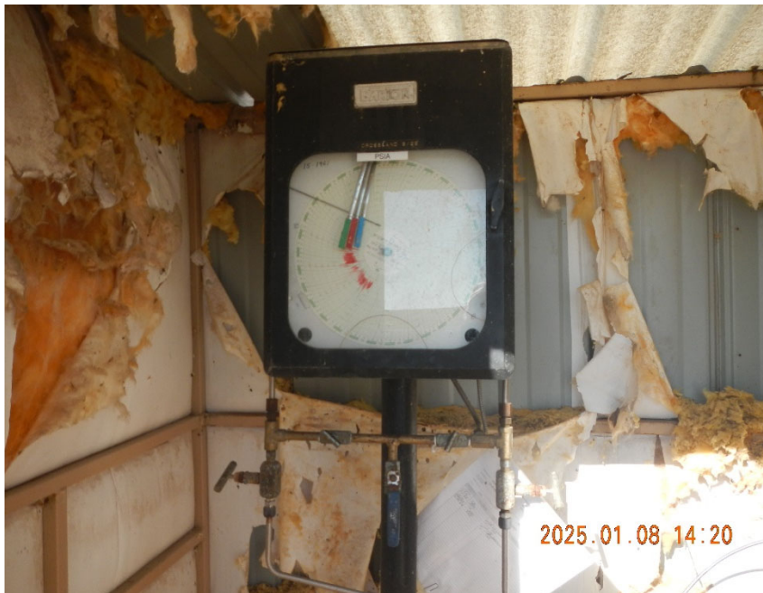
5. Gas meter inside meter shed.
