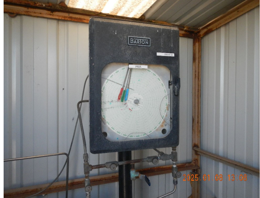
4. Gas meter inside meter shed.
