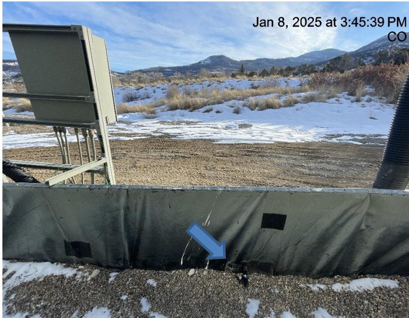
Photo # 7608 Hole in liner/liner needs maintenance
