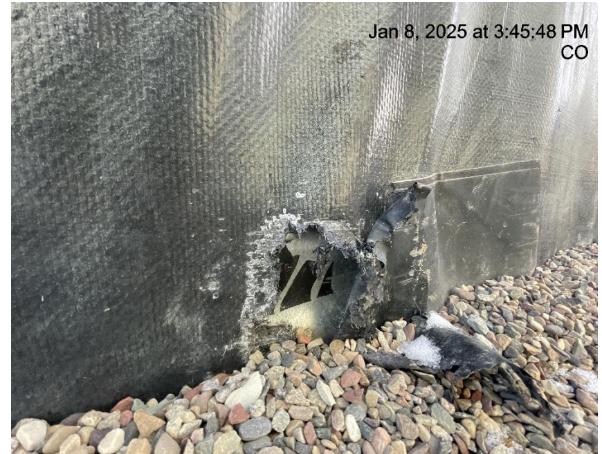
Photo # 7609 Hole in liner/liner needs maintenance
