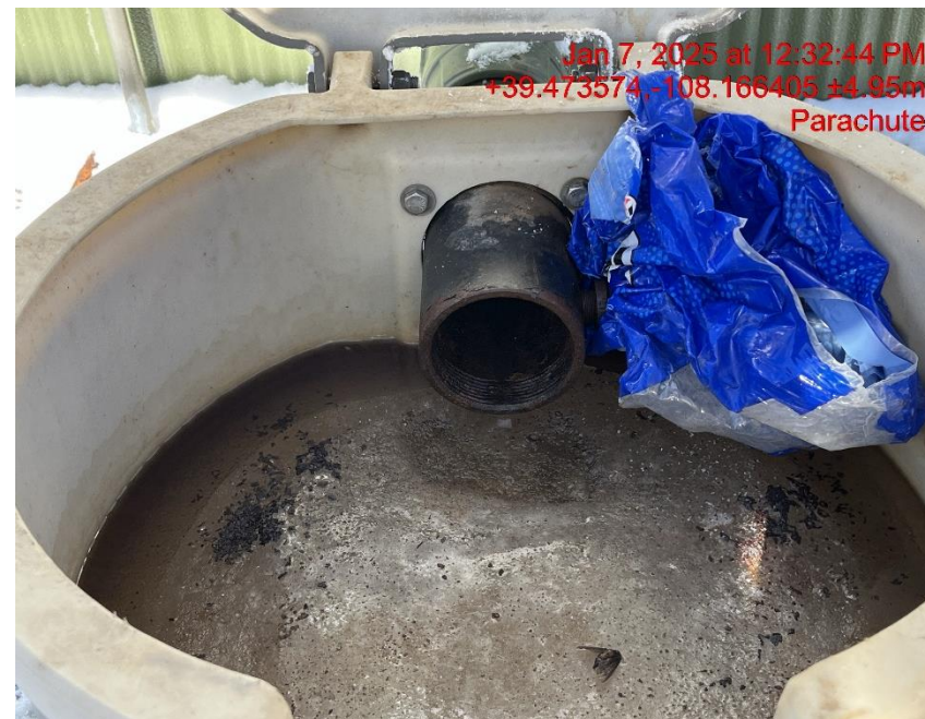
Photo # 2206 Open ended load line/Trash
