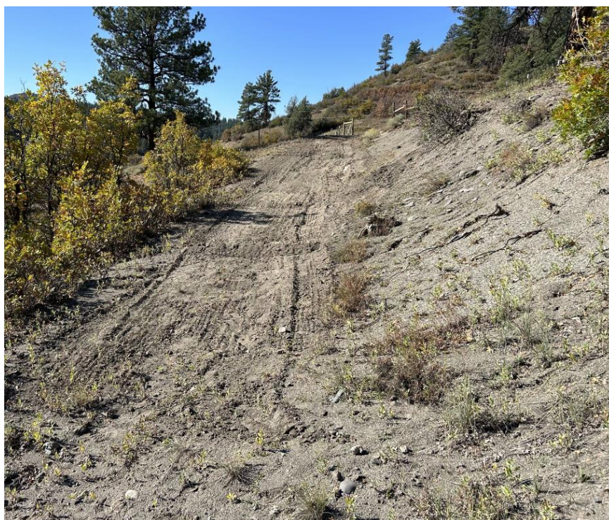
Water bars installed
