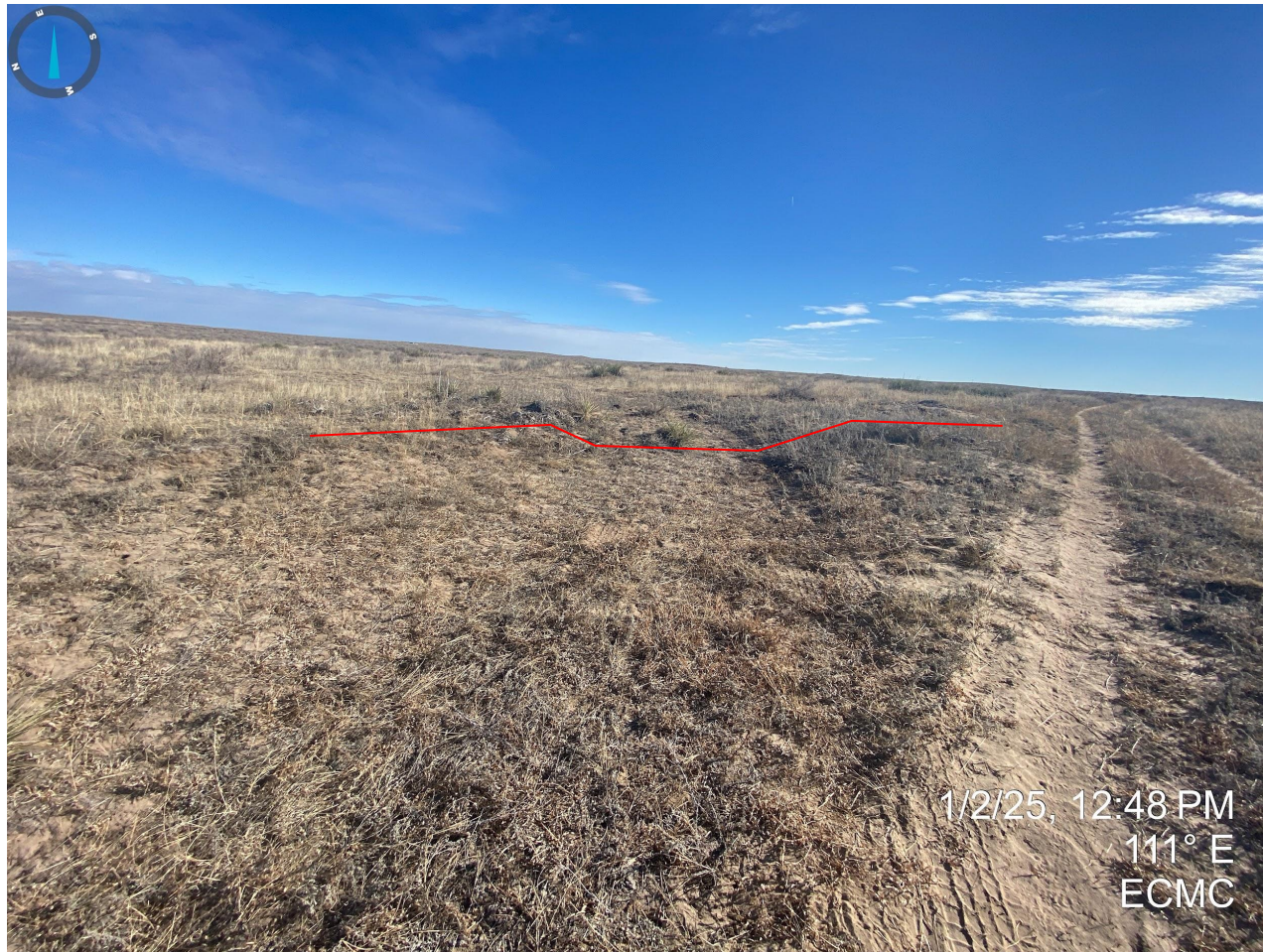
Photo 3. Access road entrance west of the former location requires additional work to contour and grade the road to match the existing grade/topography. Red line approximates current grade of access road.
