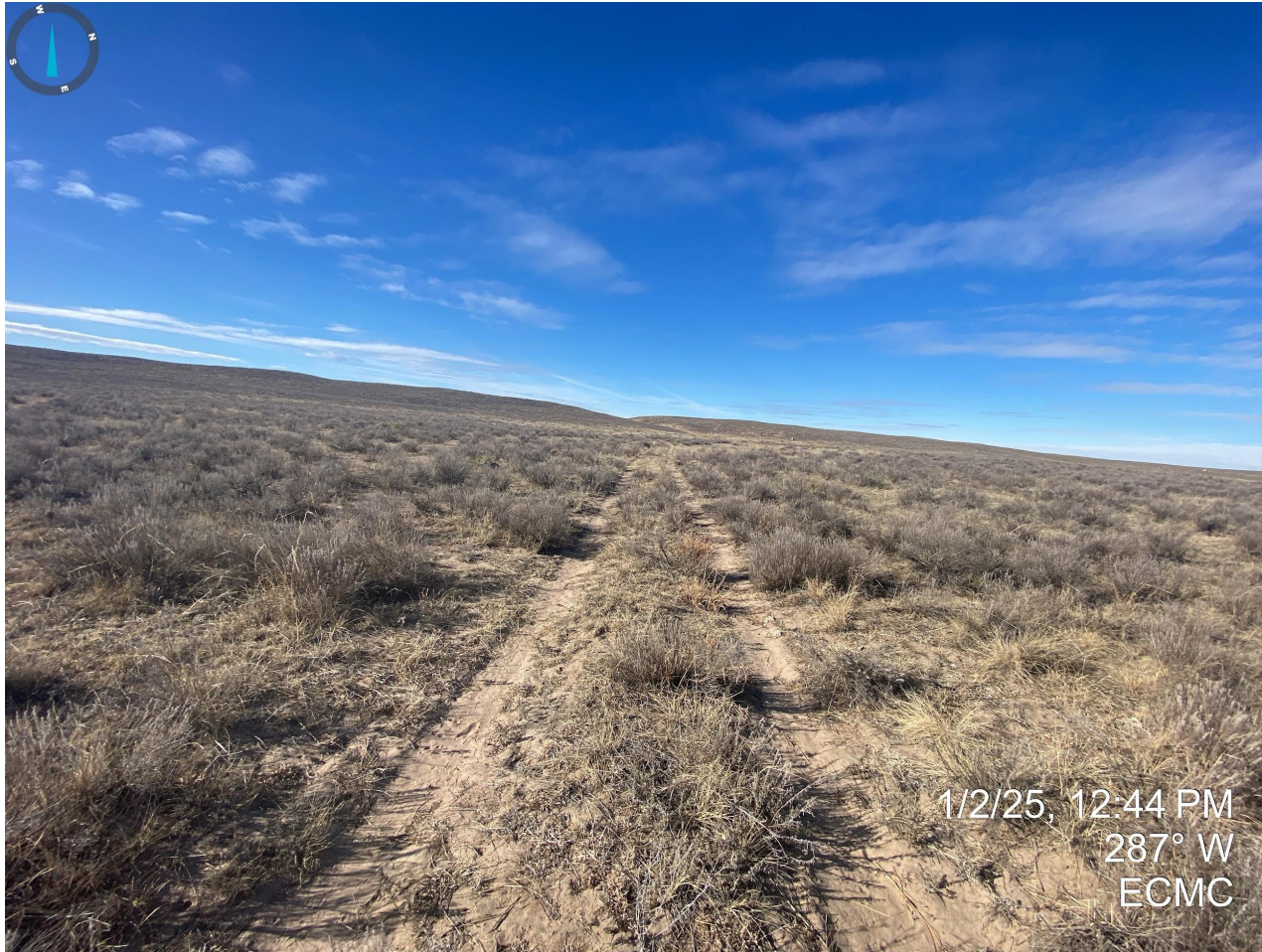
Photo 2. Portions of the access road east of the former location do not appear to have been reclaimed and require additional reclamation activities.
